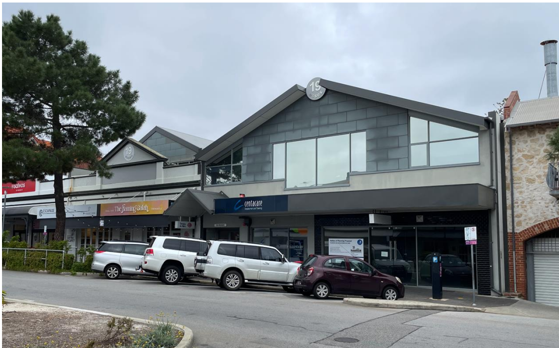
Figure 3 – Existing Street View
