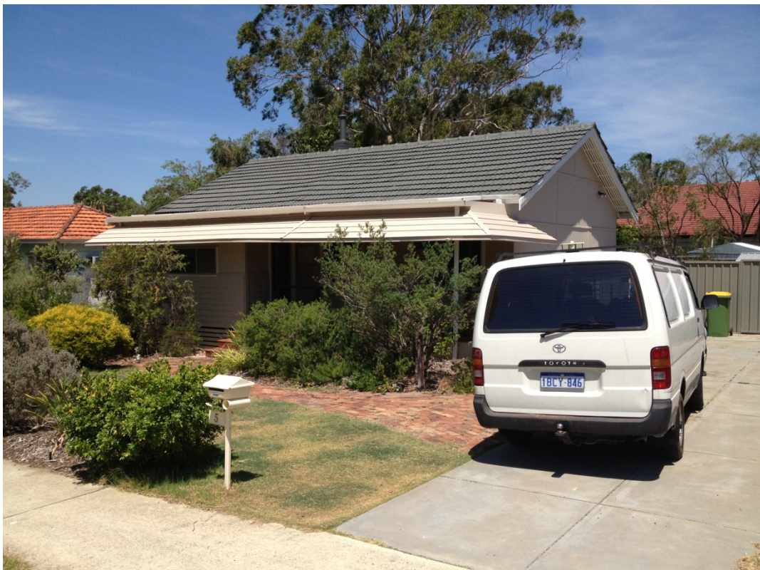
Existing dwellings at No. 5 Harwood Street, Hilton as viewed from the street.
