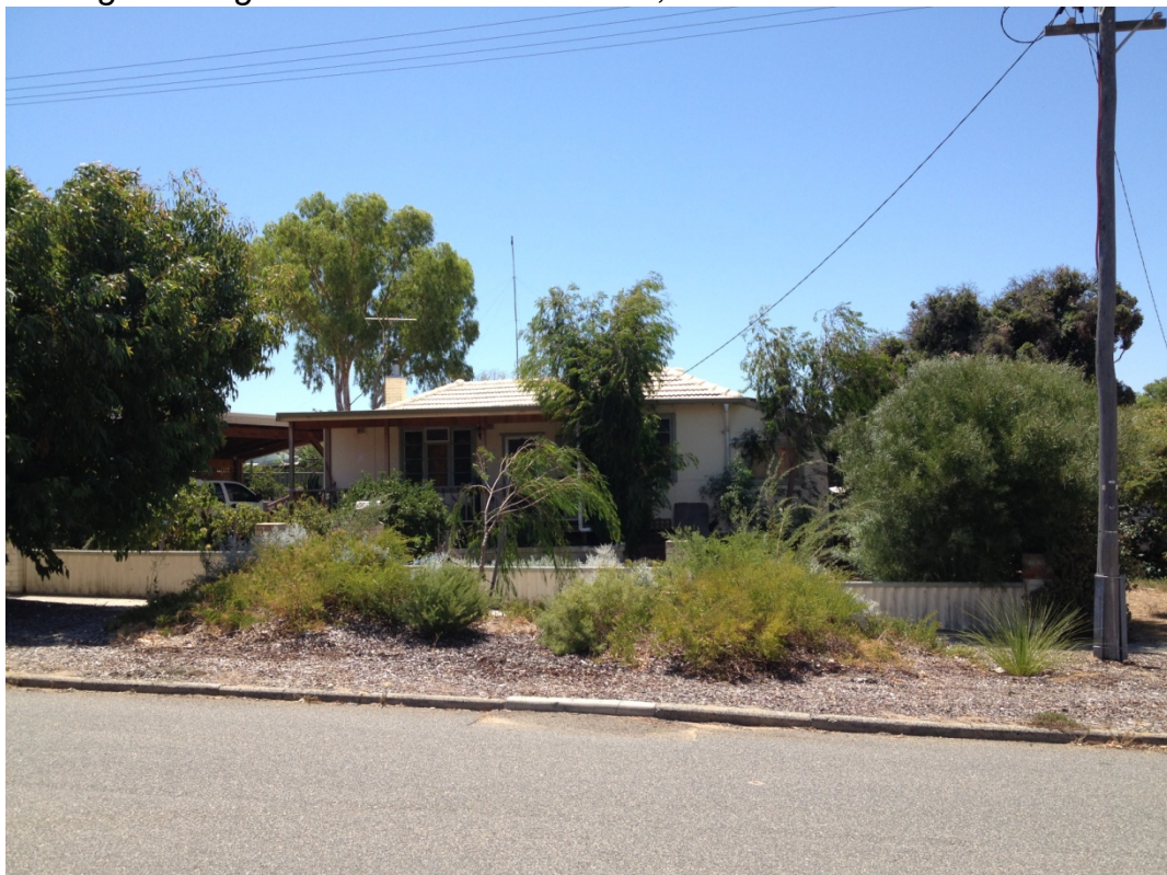
Existing dwellings at No. 4 Harwood Street, Hilton as viewed from the street in front of N. 3 Harwood Street.
