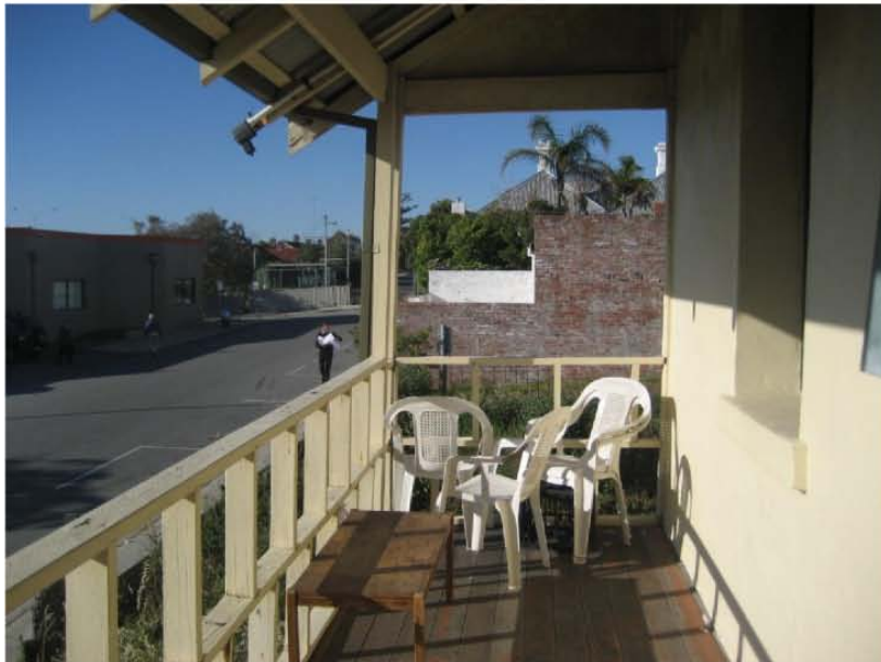
77 Quarry Street – view from verandah looking north
