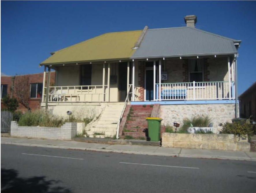
75-77 Quarry Street – front view (eastern elevation)
