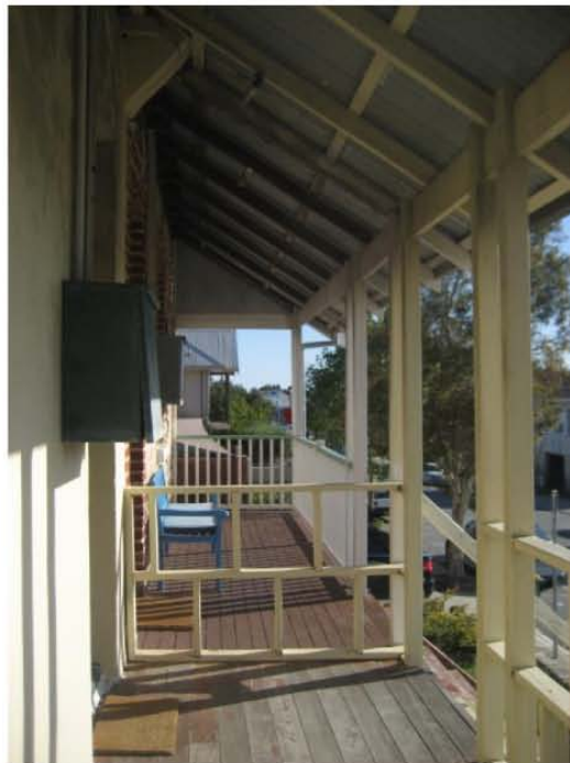
77 Quarry Street – view from verandah looking south
