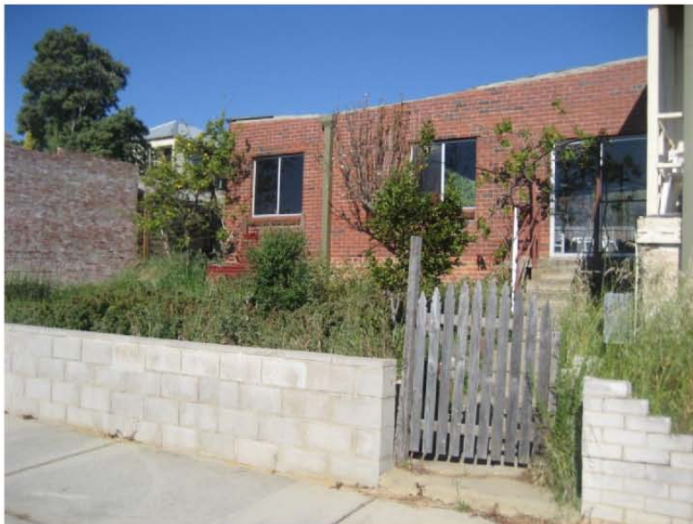
77 Quarry Street – showing additions to be demolished
