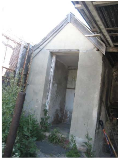
77 Quarry St – rear WC
