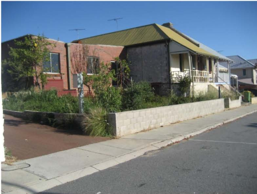
2 Hickory Street – showing front awning over window
