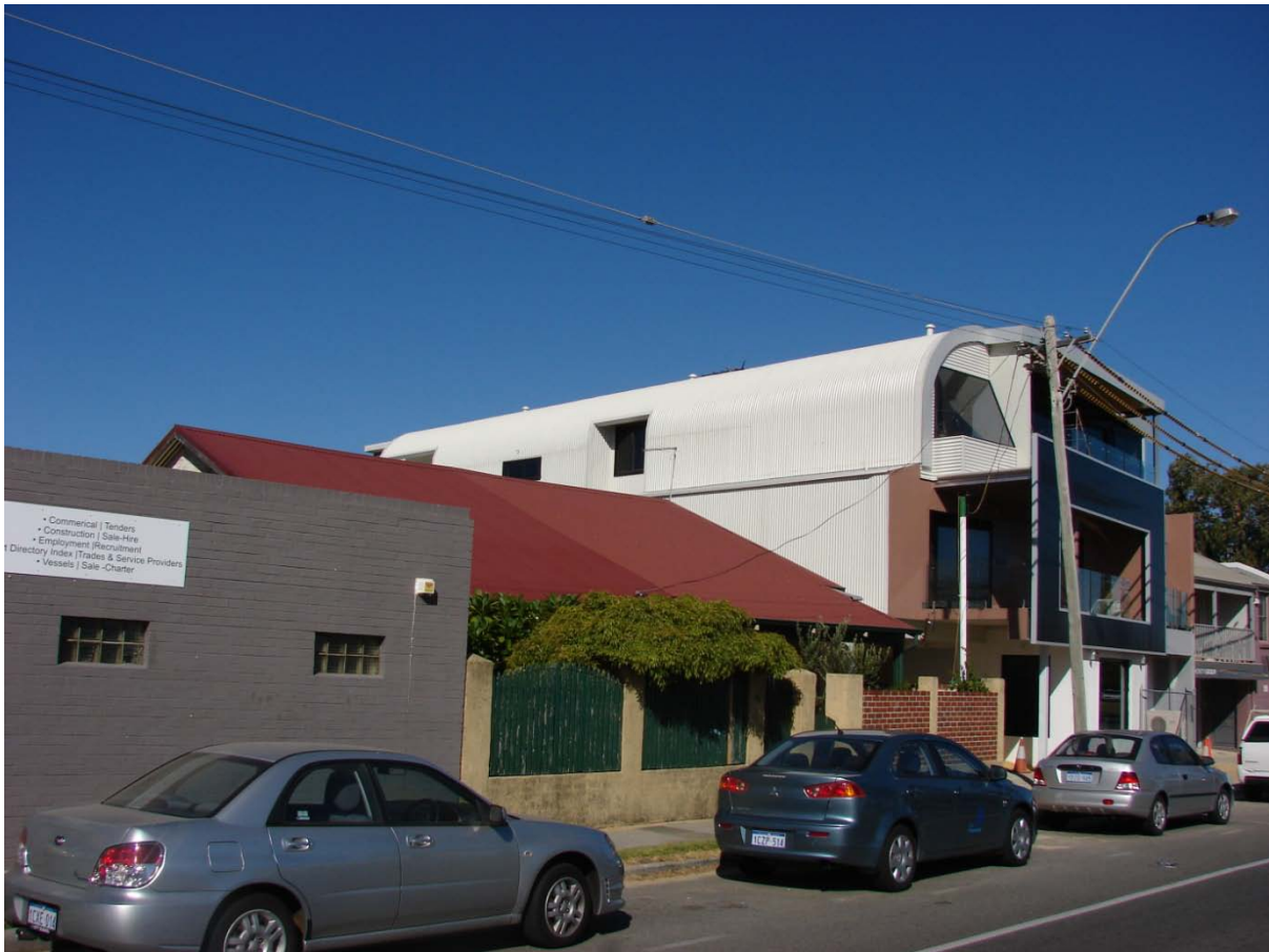
Photograph 7 – refer to comments made on Item No S2 of report.
