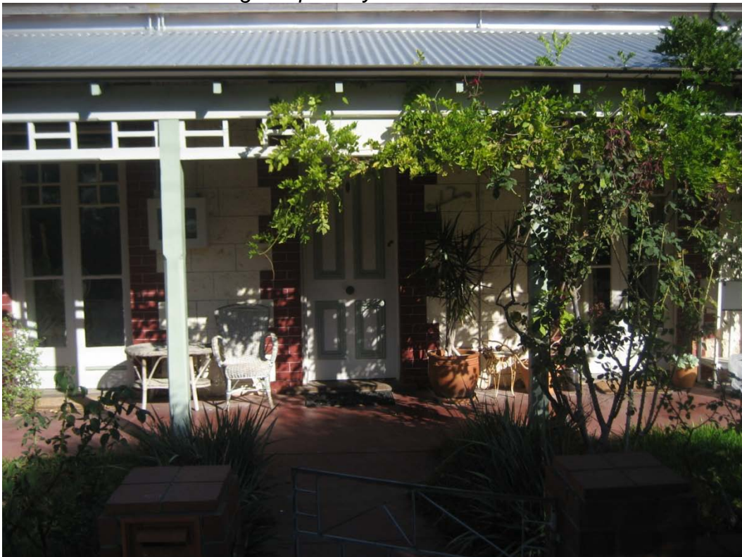
View of the existing verandah and front facade from Ainslie Street.
