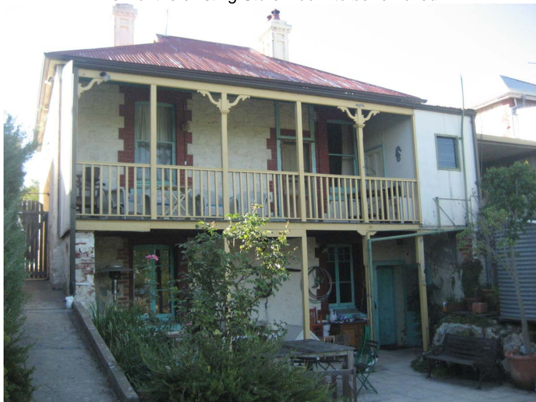
View of the rear of the existing Single House (showing the Ground Level and Undercroft).
