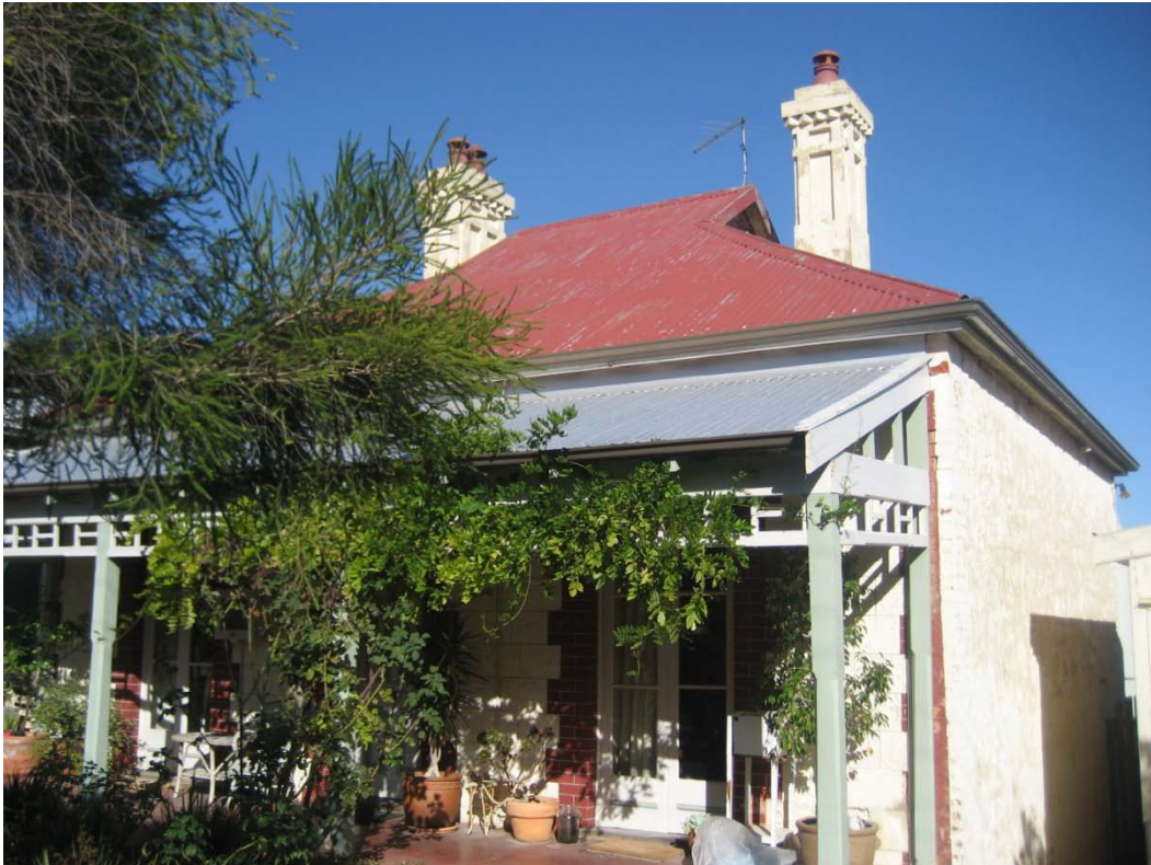
View of the existing Single House from Ainslie Street.
