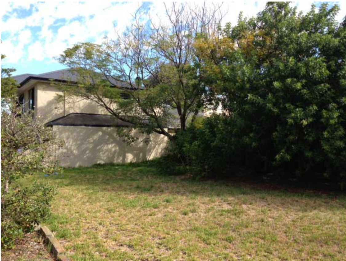
Boundary wall – 1 Amherst Street (southern portion of site)
