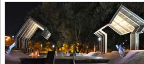
FEATURE LIGHTING, WODEN SKATEPARK
