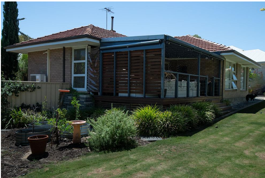
Photo 2: View of front of No.60 Chadwick Street, from behind front boundary fence / shrubs
