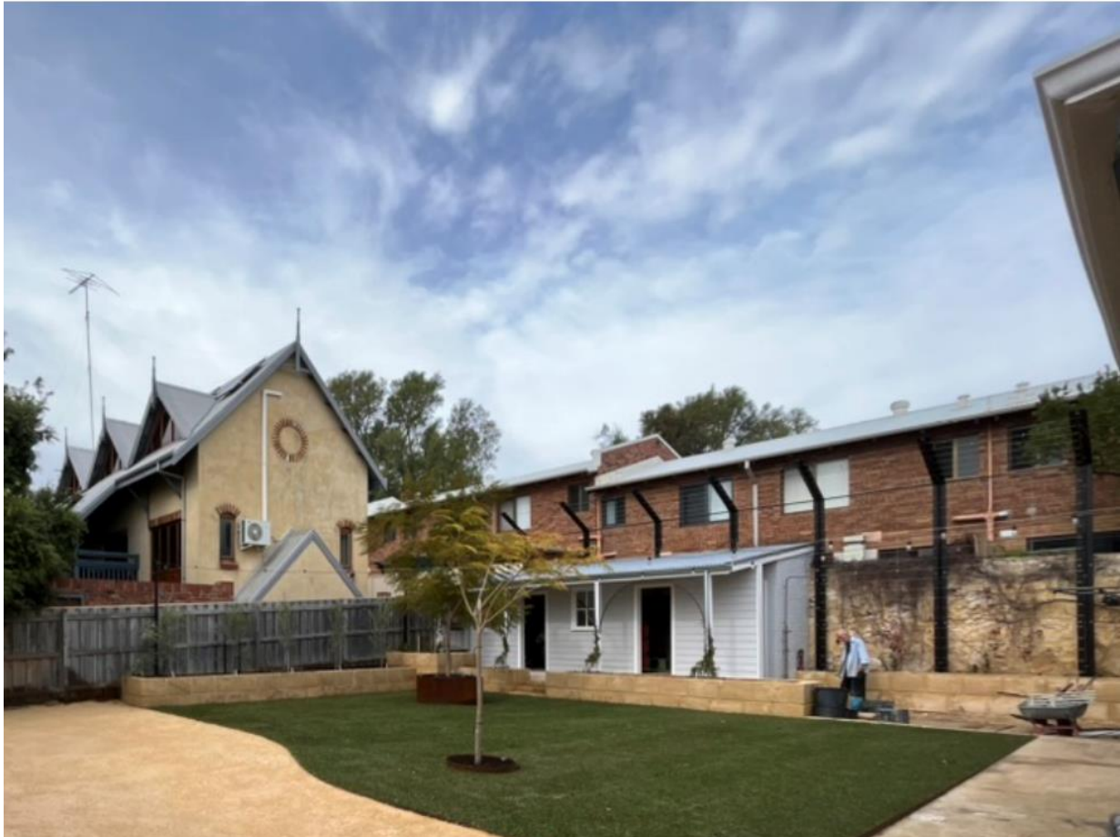
Figure 1. Unauthorised external fixture (permeable, open framework screening structure) along the southern boundary, toward the rear of subject site.
