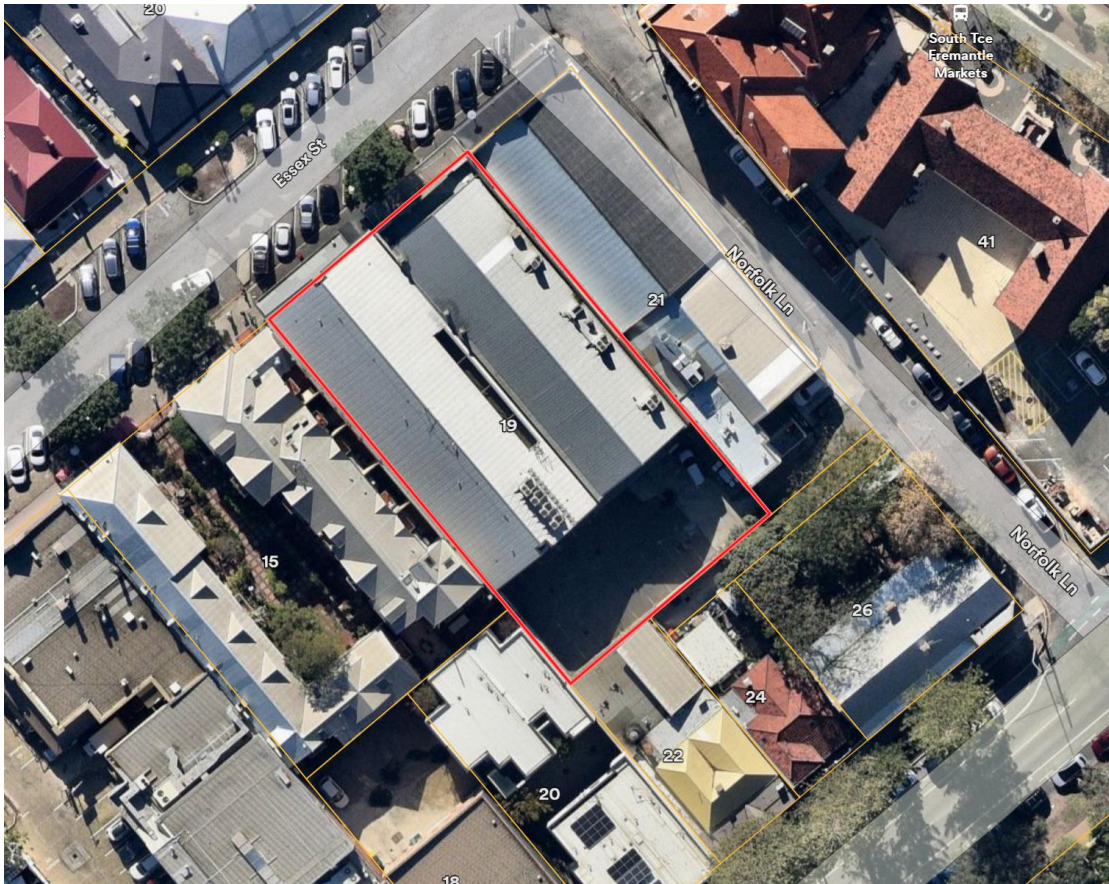
Figure 2 – Site Aerial Image
