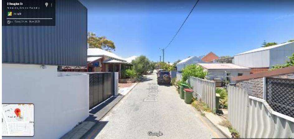
Douglas Street, Fremantle - no footpath possible due to width:
