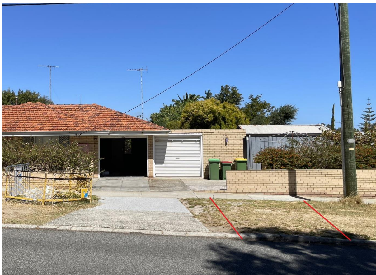
Figure 8 – Existing crossover and the approximate location of the proposed crossover marked in red.
