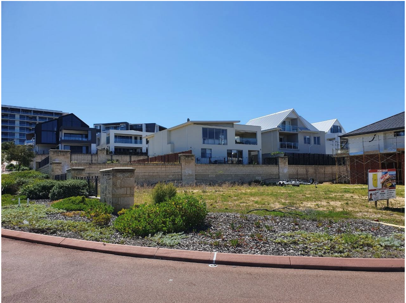
Photo 1: Subject site shown from Westmeath Street showing surrounding similar development at 38, 43 and 45 Mathieson Street.
