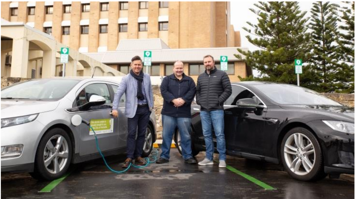
Figure 3 Solar powered LED lights and electric vehicle charges at Cappuccino Strip car park
