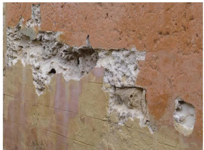
*Two examples of the decay caused by impermeable cement mortar, which forces the limestone walls to dry through the stones. Salts accumulate in the stones which erode away, leaving the mortar standing proud. It's much cheaper and easier to replace mortar (repointing) than it is to replace stone.*
