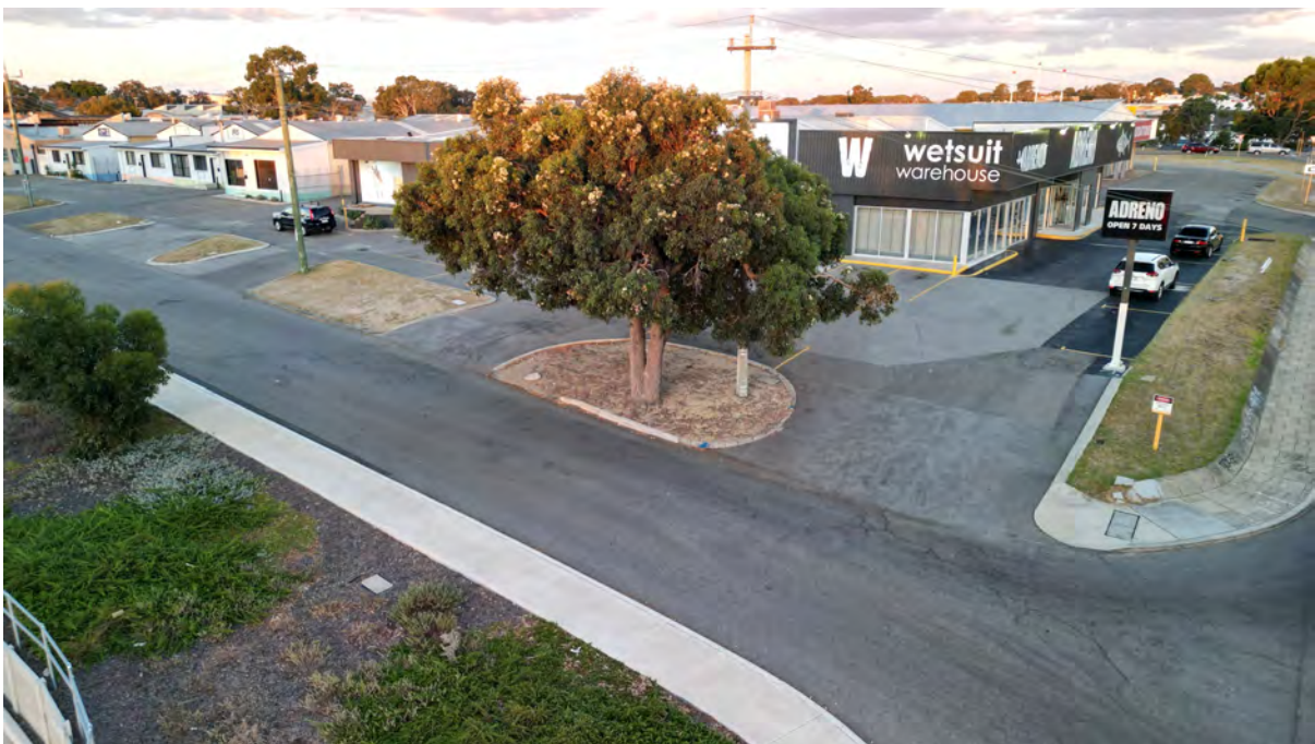
Figure 4 - Existing condition - North East view.
