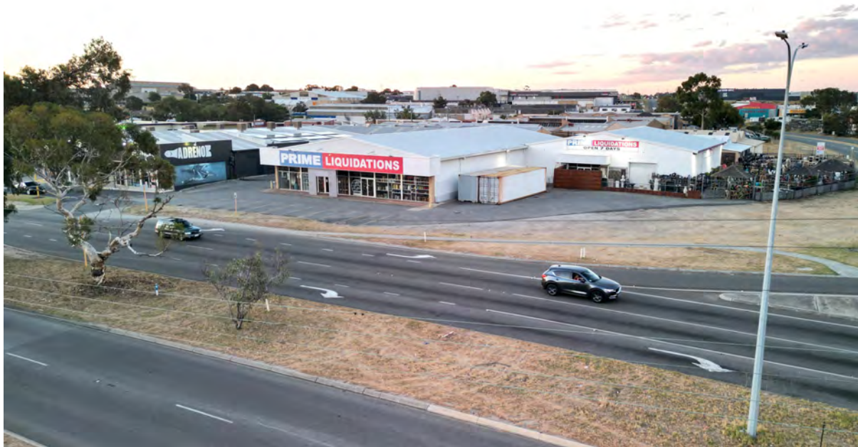
Figure 2 - Existing condition - North West view.
