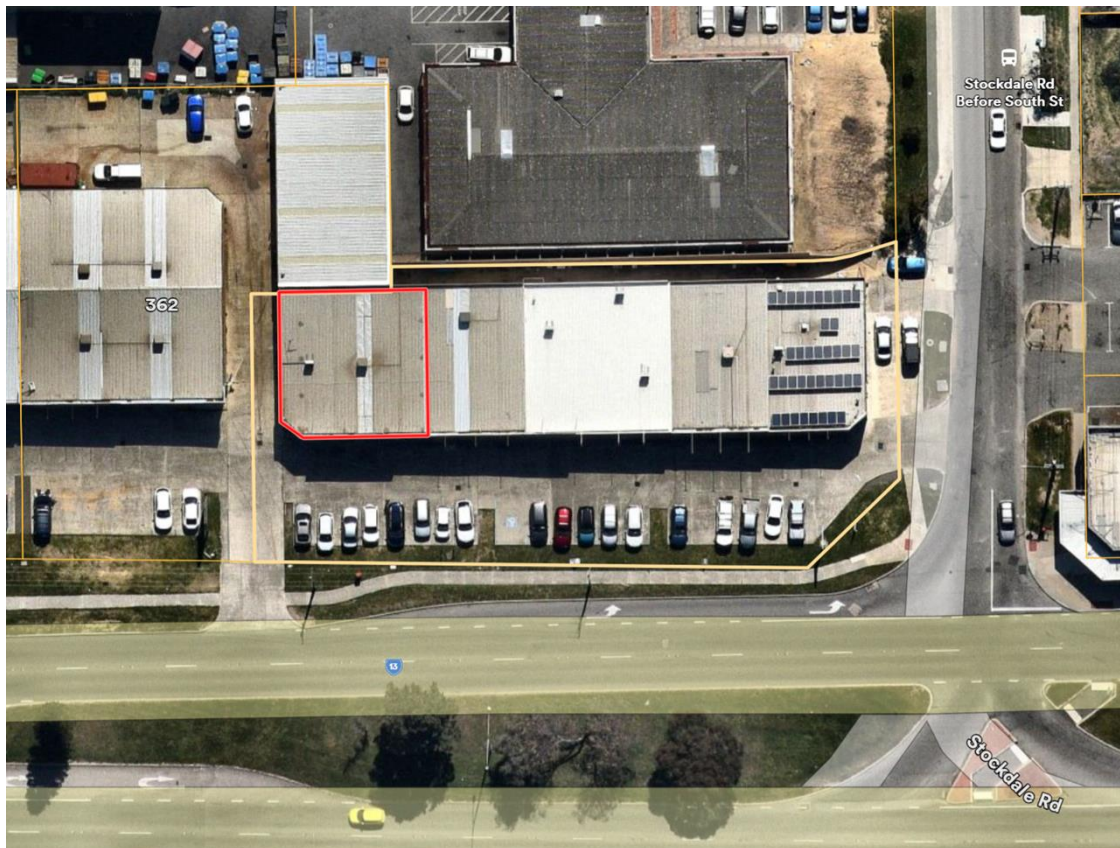
Figure 2 – Premises 1/364 South Street outlined in red.
