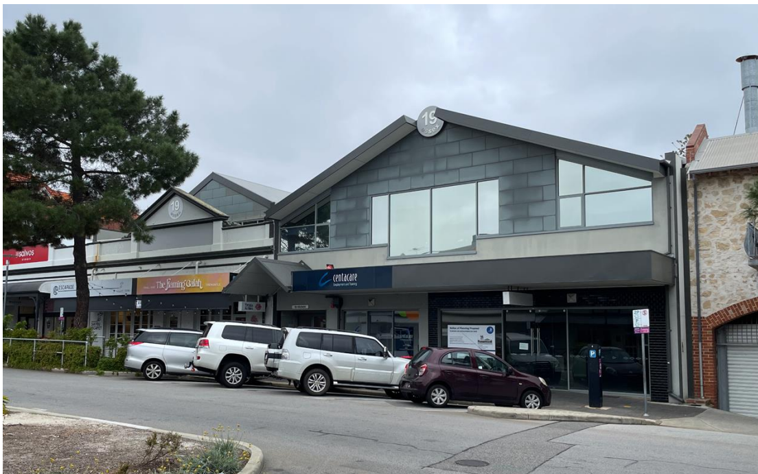
Figure 3 – Existing Street View
