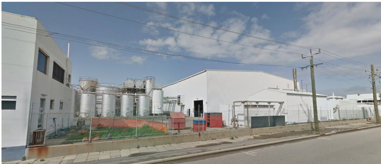
Photo 1 – Industrial tanks and sheds proposed for demolition on western side of Bracks Street,
