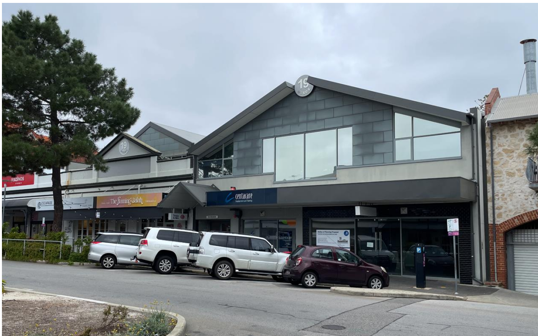
Figure 3 – Existing Street View
