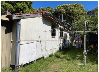
West elevation with enclosed back verandah and attached steel framed patio roof.
