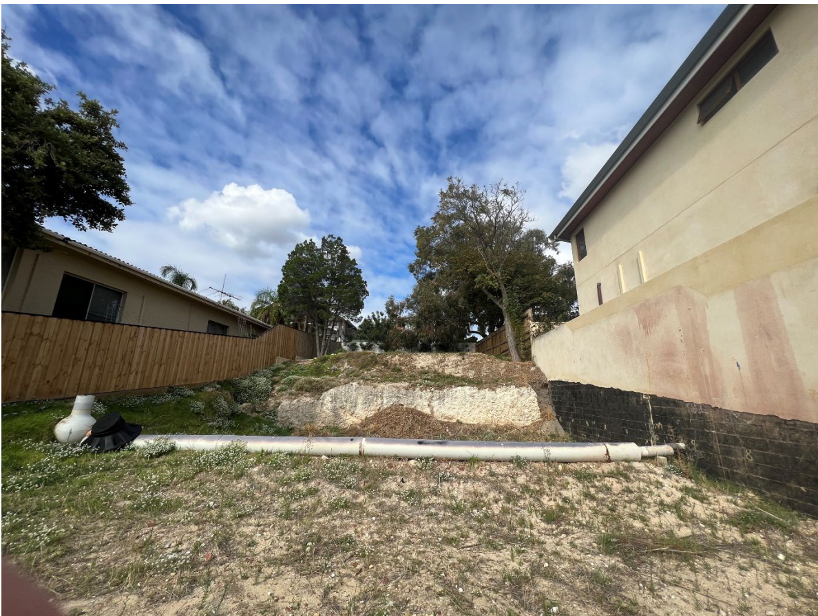
Figure 1 – Photo of the site as viewed from Alfred Road
