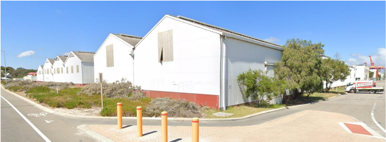
Photo 3 – Existing buildings on site proposed for demolition (viewed from Walter Place)
