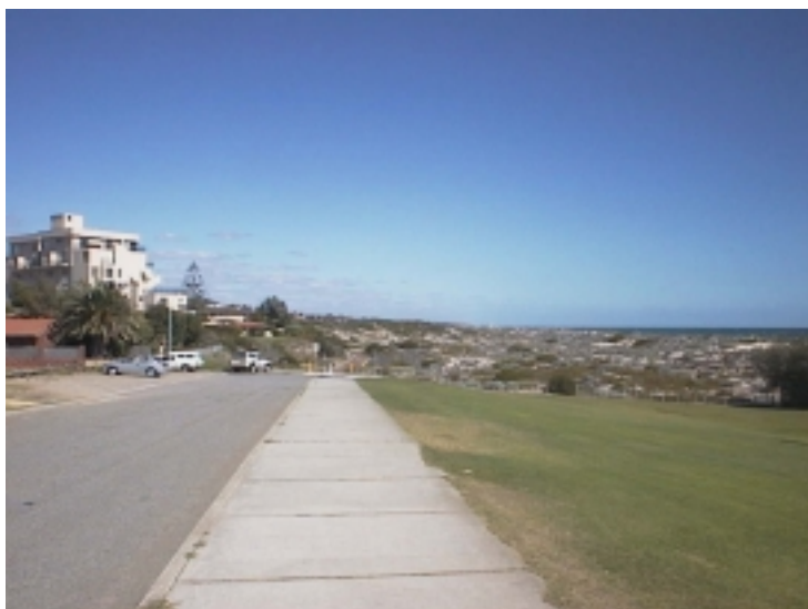
Photograph 1: Showing infrastructure, housing and recreational facilities are set well back (approximately 200 metres from the beach at Scarborough Beach).
