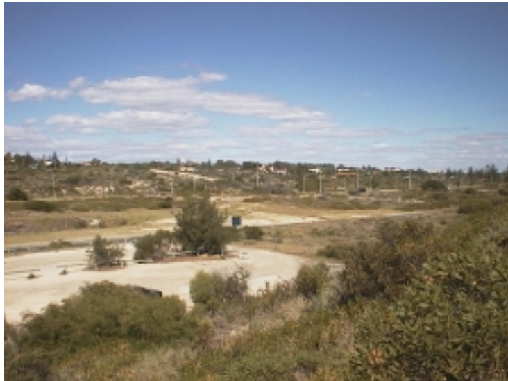
Photograph 7: Example of a nodal car park set back behind the dunes, South Scarborough. Natural surface to minimise visual impact of the car park and allow infiltration of rainfall.
