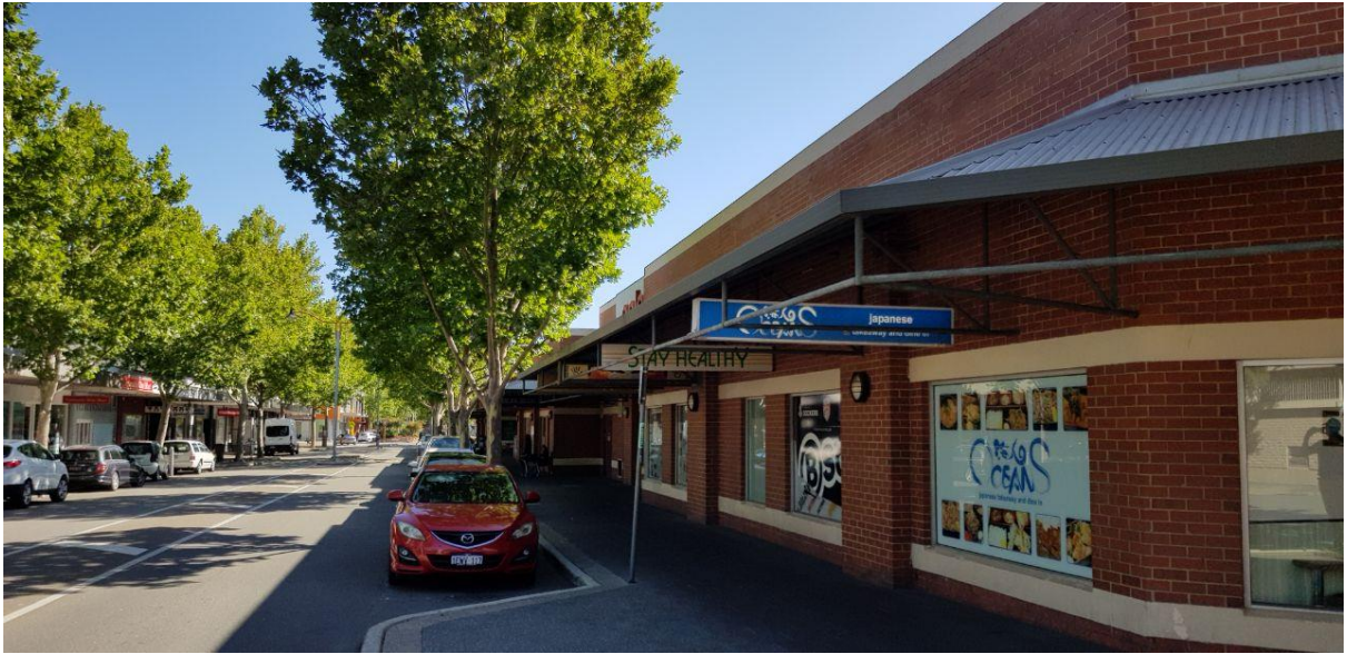
Figure 9: Existing shopping centre from Cantonment Street
