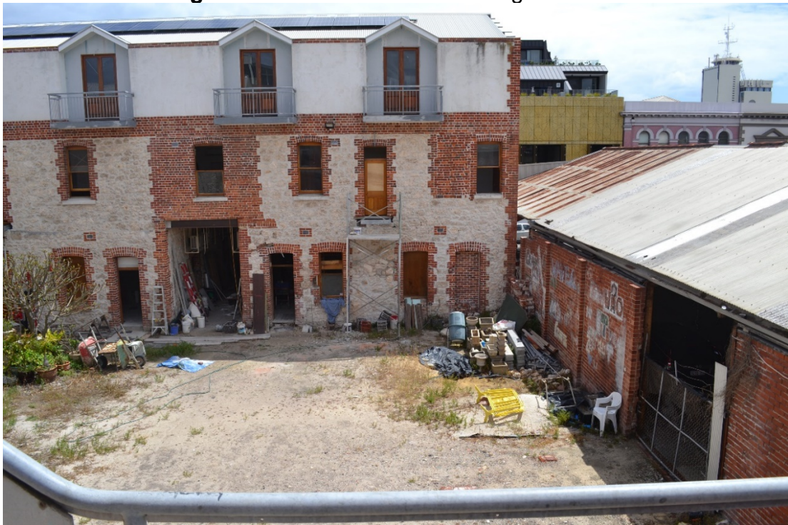
Image 4: view from staircase looking west
