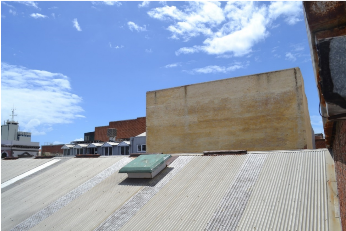
Image 5: view from staircase looking north-west
