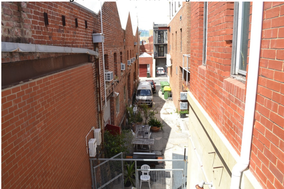
Image 6: view from staircase towards Pakenham St via Right-of-Way (looking east)
