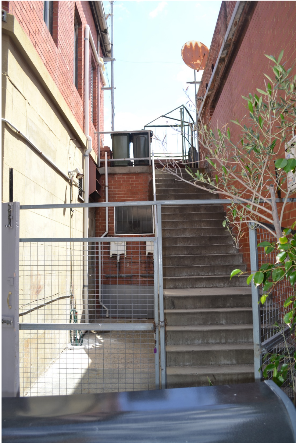
Image 8: view of staircase from Right-of-Way looking west.
