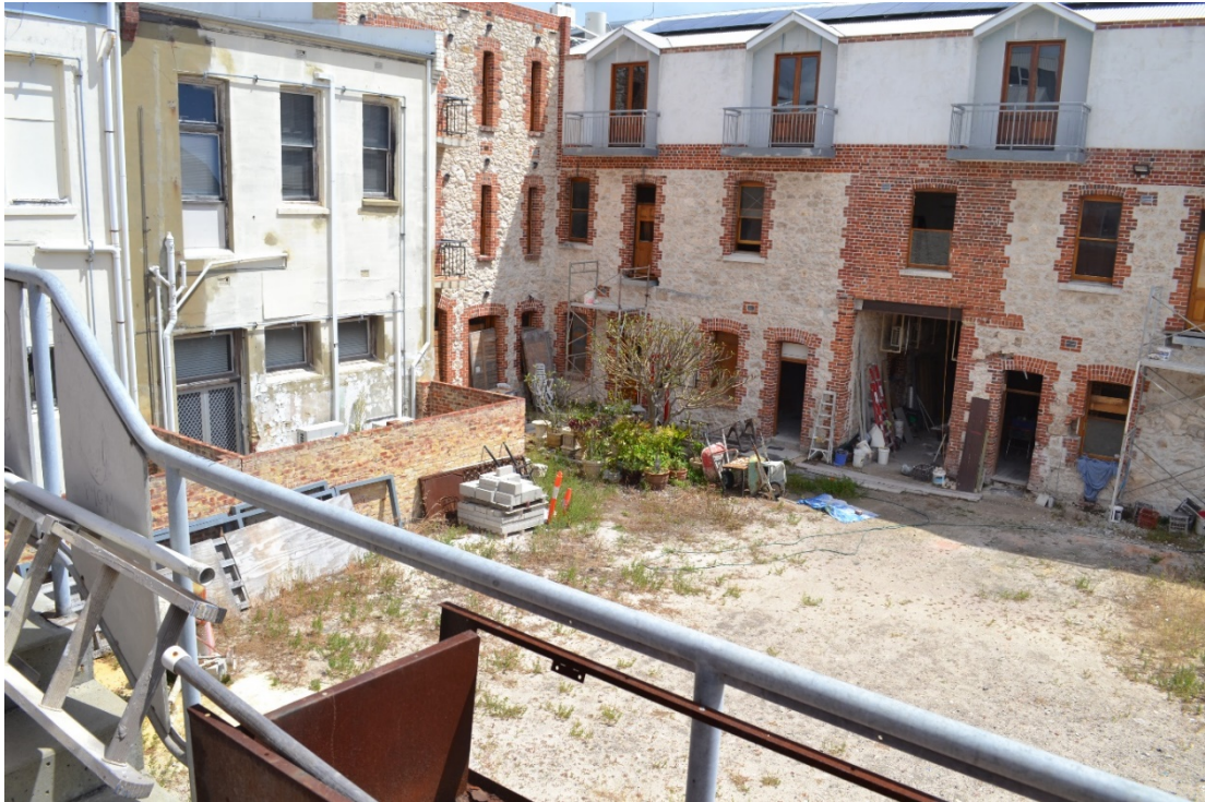
Image 3: view from staircase looking south-west
