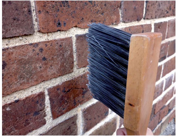
A stiff-bristled churn brush being used to tamp the new work, compacting the mortar, exposing the sand grains, and producing an aged appearance. (Photograph: David Young)
