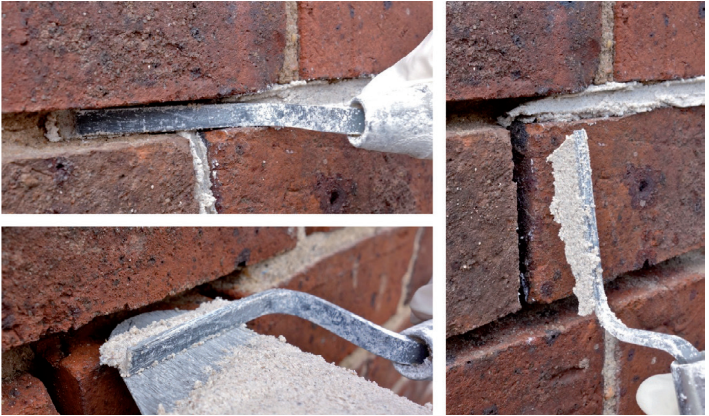
Caulking or finger trowels are used to place mortar into the back of raked-out joints. Different size trowels are needed for different joint widths. With care, no mortar need be smeared on the face of the bricks or stones. (Photographs: David Young)
