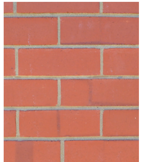
Modern brickwork with rolled or bucket handle joints c. 1970s.
