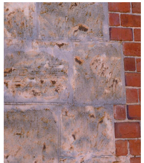
Remnants of original raised ribbon pointing to limestone wall.
