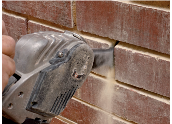
An oscillating blade tool can be used to cut out soft to moderately hard joints without damaging the masonry units. (Photograph: David Young)
