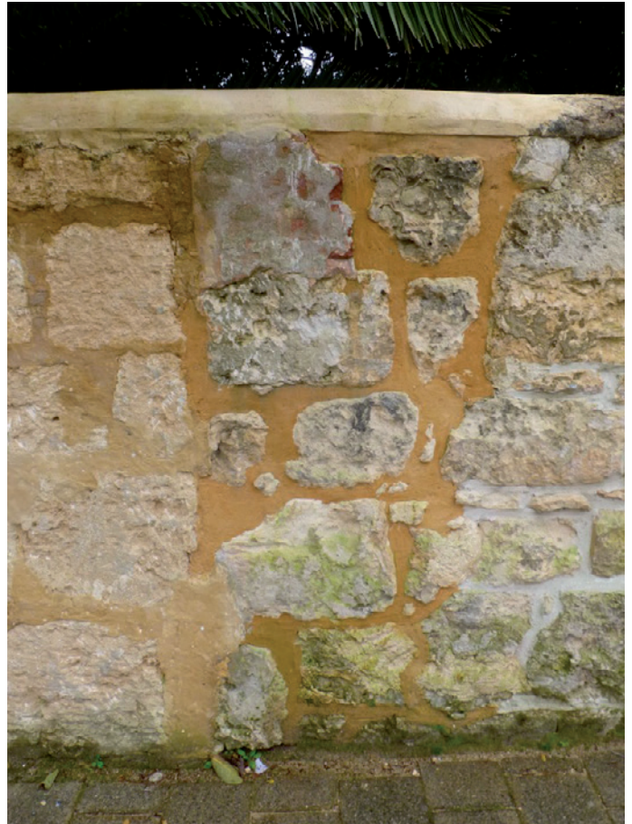
Recently completed repointing to limestone garden wall dating from 1850s but with a number of modifications made in the 1890s. Different pointing styles and colours were identified from the different eras of development and replicated to retain the evidence of change. All repointing used lime mortars and the colour variation is due to the type of sand used in the mix. It is thought that the earliest section of wall (left) used sand dug up on site whereas the later sections (central and right) were sourced from local quarries.
