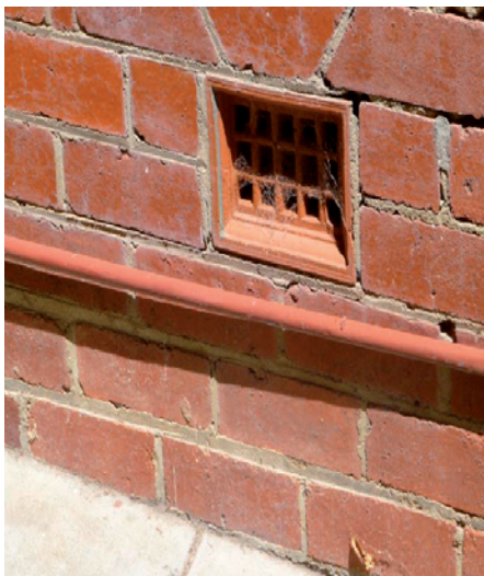
Traditional Western Australian cut and struck (or overhand struck) pointing.
