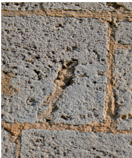
Remnant of original joint with mortar coloured with 'Spearwood Red' sand to school building c. 1900.
