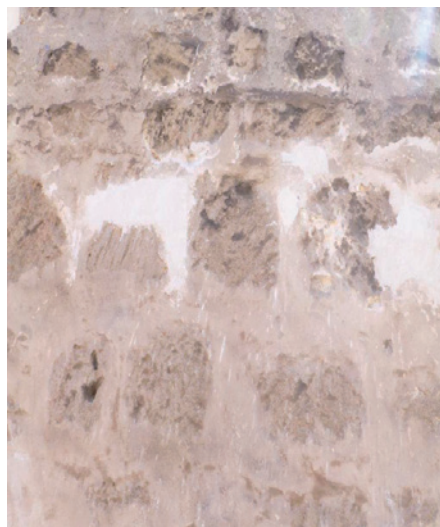
Original flush pointing to side wall of house c. 1890s.
