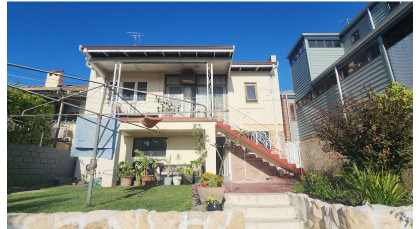
HOUSE PHOTO SHOWING EXISTING BALCONY TO BE REPLACED.
