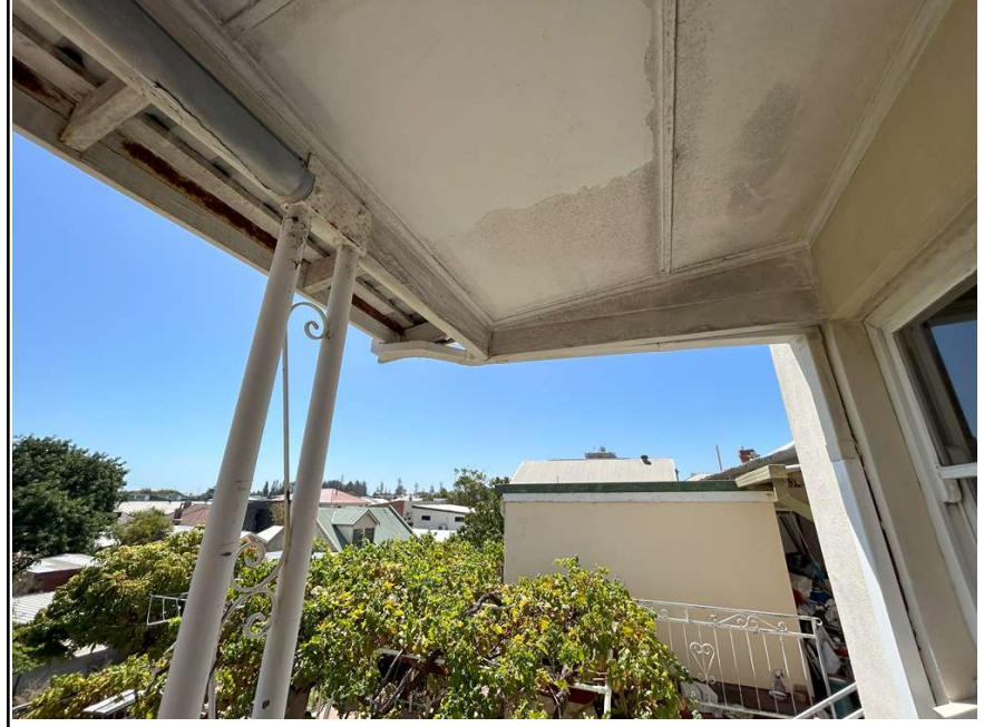
VIEW FROM BALCONY OVERLOOKING NORTH SIDE
