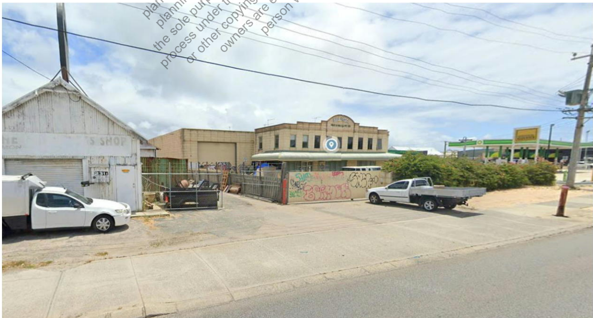
Figure 2: Streetscape Looking North West
