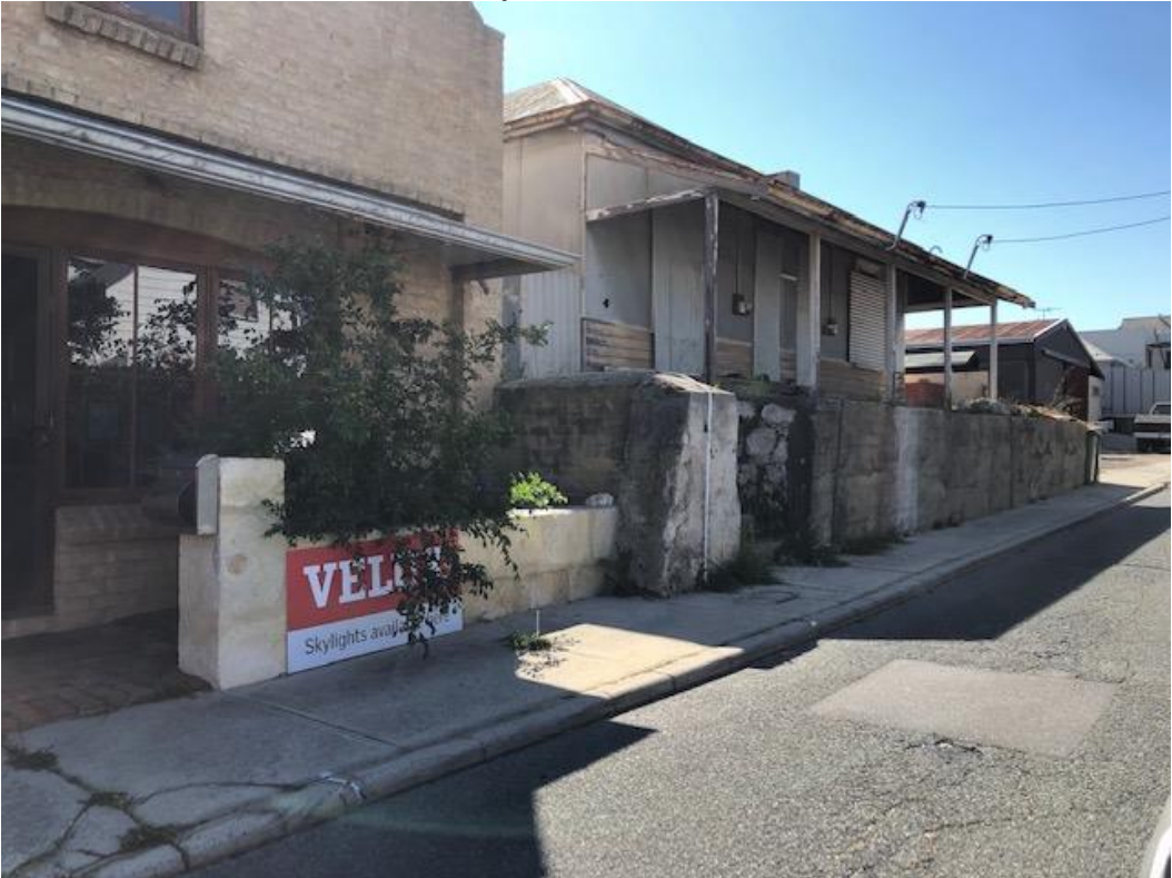
Photo 3 – South eastern view of the subject site
