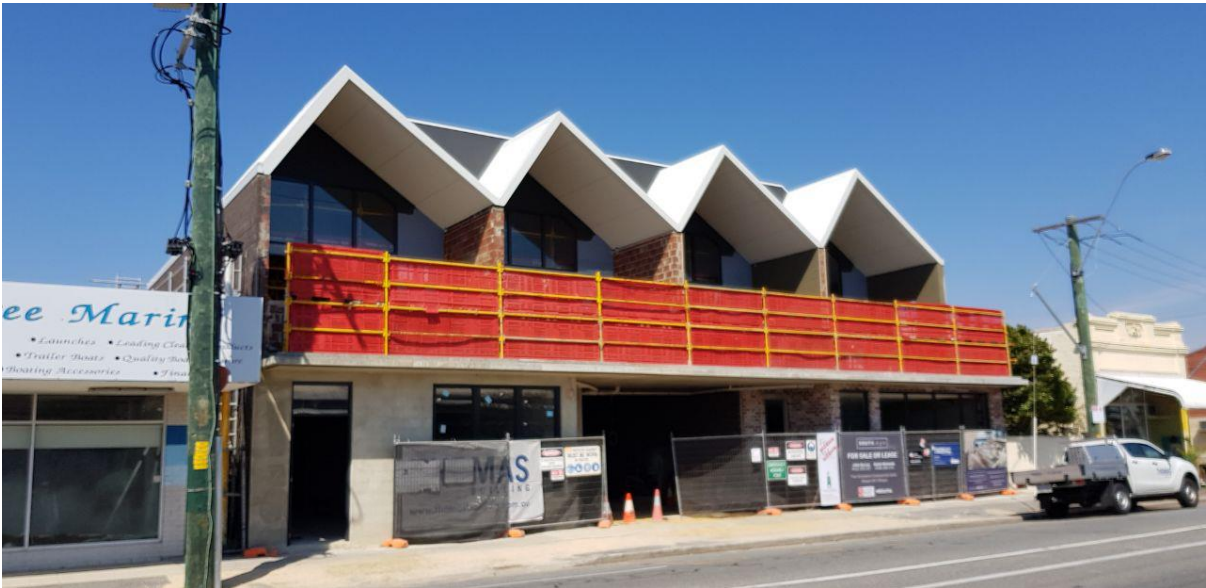
Photo 1: Site from South Terrace
