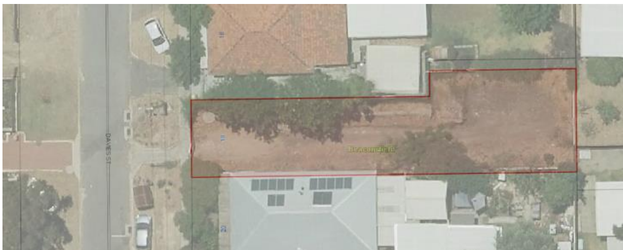
Image: Drainage Sump, 18 Davies Street Beaconsfield.
