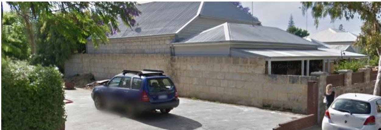
Figure 2: Adjoining boundary wall
