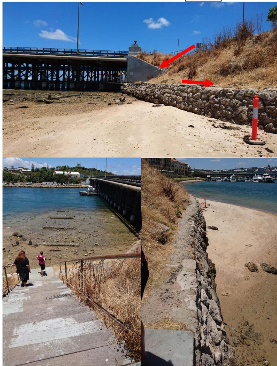
Figure 2-10 Existing concrete step.
