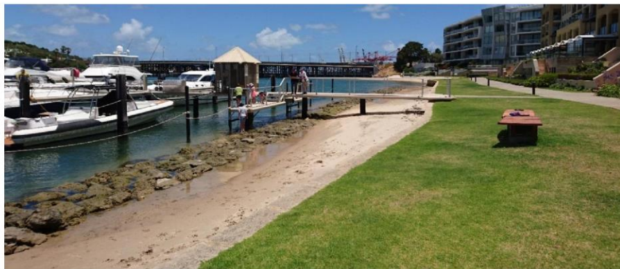
Figure 2-8 Boat pens and scour protection rock wall east to the project site.
