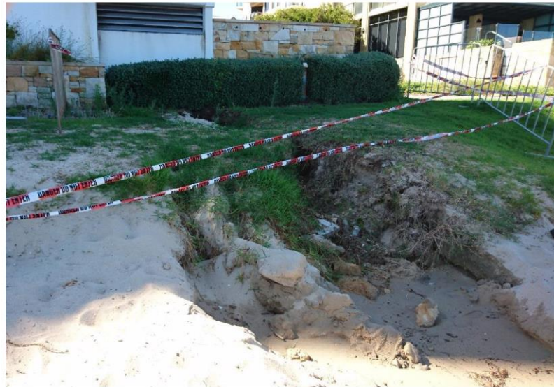
Figure 2-19 Foreshore erosion after rainfall event on the 9 February 2017.
