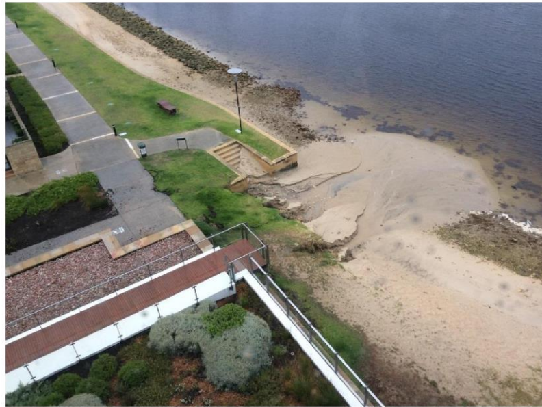
Figure 2-20 Photo taken on the 10/02/2017 provided by a resident of the Rivershores Apartments.
