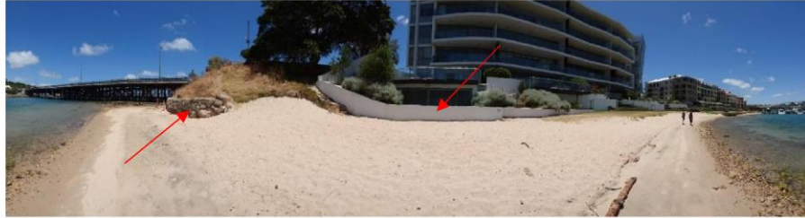
Figure 2-7 Panorama view of the project site, with the concrete retaining wall and rock retaining wall indicated.
