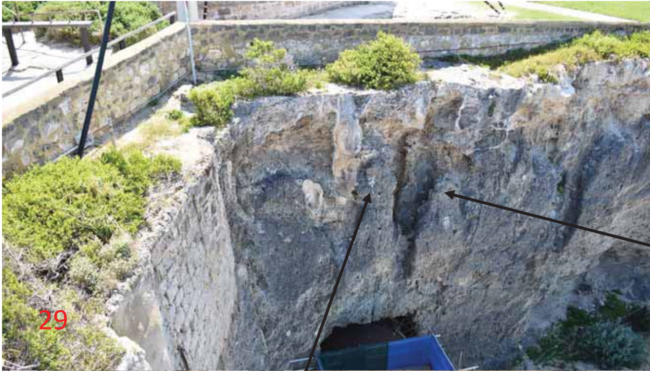
Area 7 – Vertical Face over western tunnel portal
