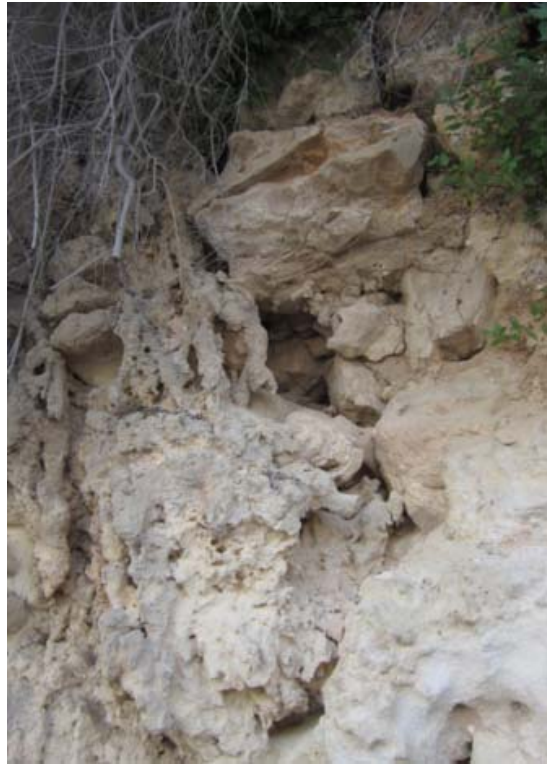
the barrier wall on top of the cliff which is in a poor state of repair.
