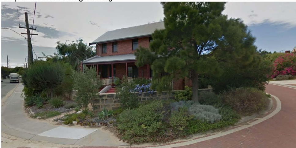
Southern neighbouring site – No.2 Binns Court, North Fremantle
