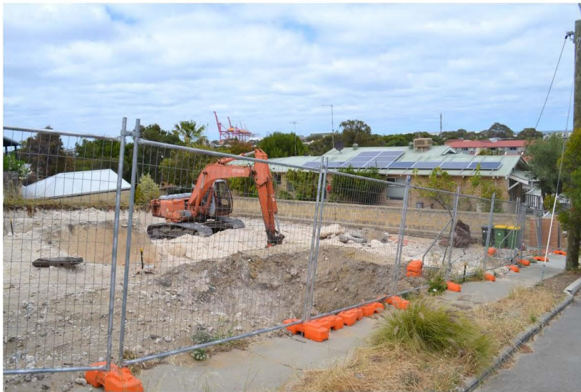
Photo 2: Streetscape looking towards the west
