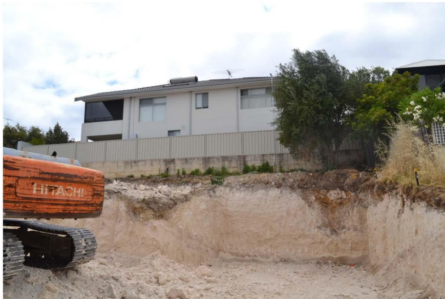
Photo 6: Interior of lot towards east (6 Letitia Rd)
