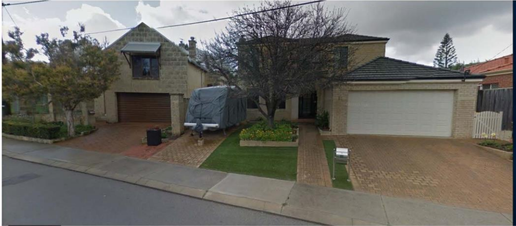
Two neighbouring northern sites (No. 85 and 87 Thompson Street, North Fremantle)
