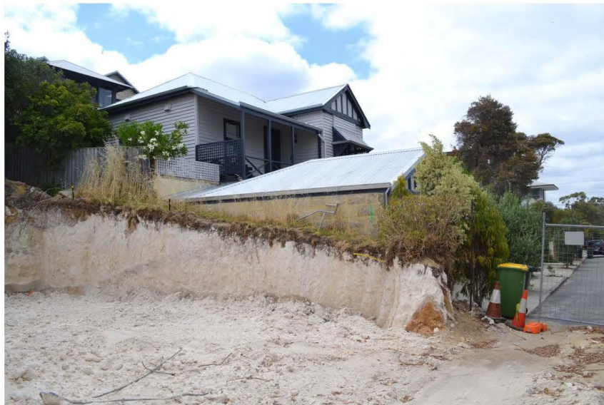
Photo 5: Interior of lot towards rear (31 Herbert Street)
