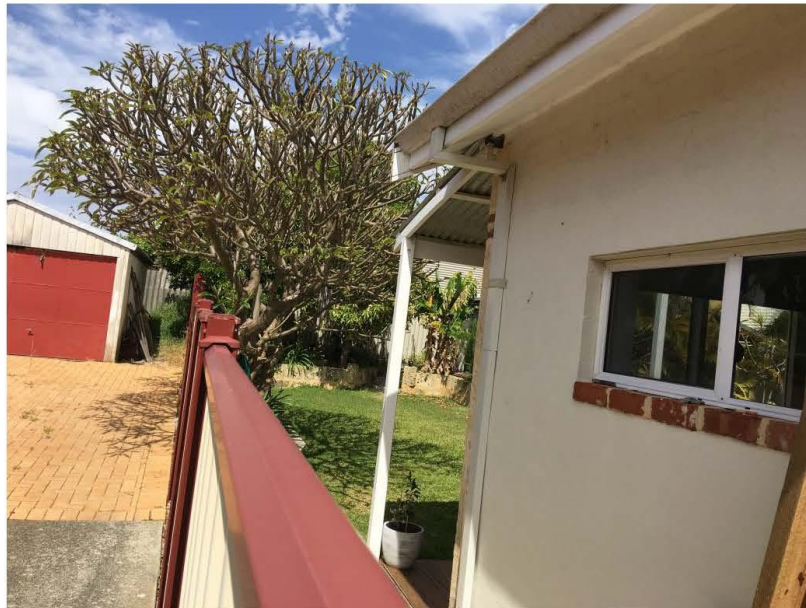
Photo 3: View from southern dividing fence into adjoining lot.
