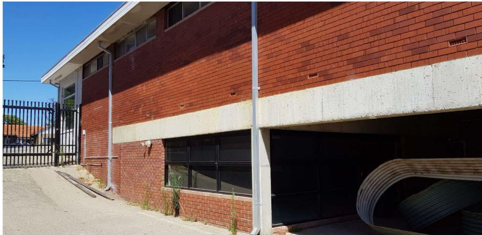
View of side of existing building
