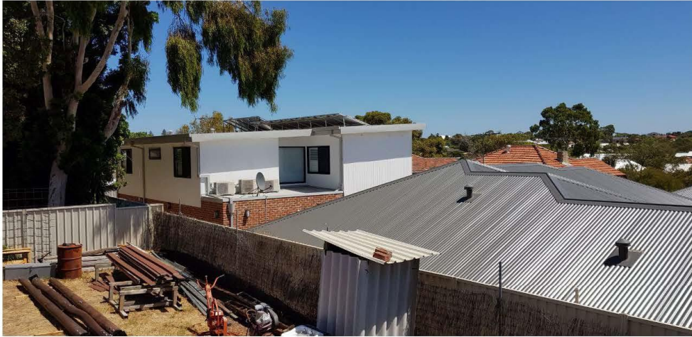
View from rear stair facing north west
