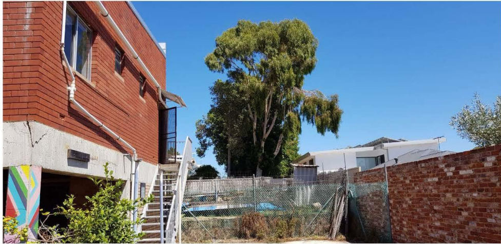
View of adjoining rear yard and rear of building facing west
