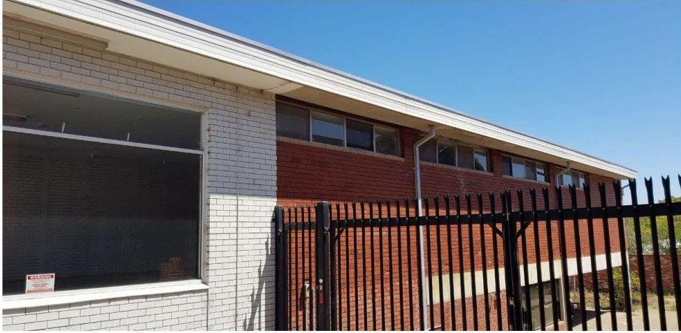
Side of existing building
