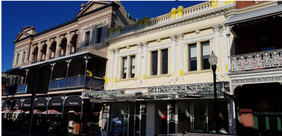
Photo 2: View of site from High Street
