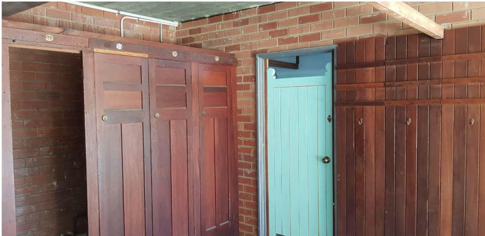
View of existing store area and building access
