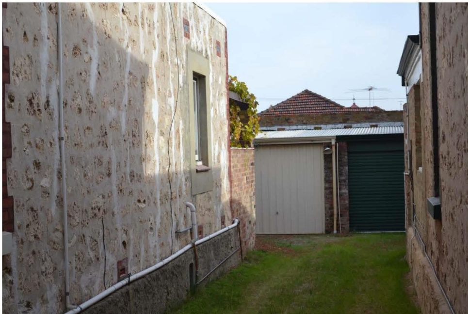
Photo 2: View down existing driveway between No. 53 and No. 51
