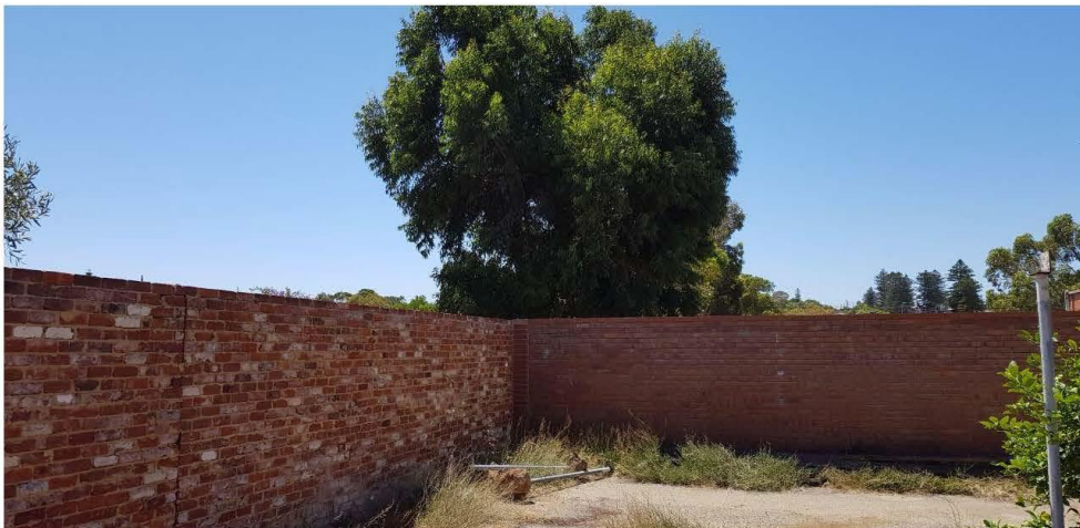
View of rear yard facing north east
