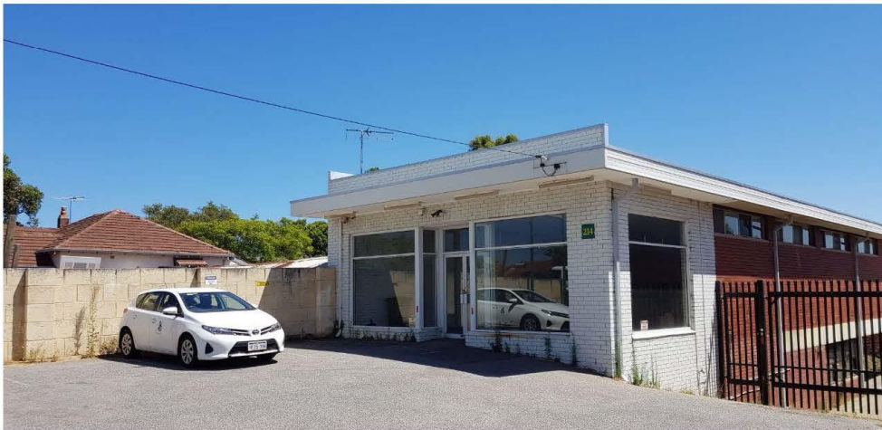
Front of existing building
