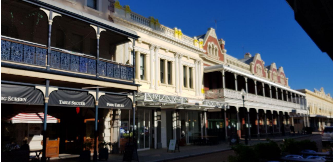
Photo 1: View of site from High Street
