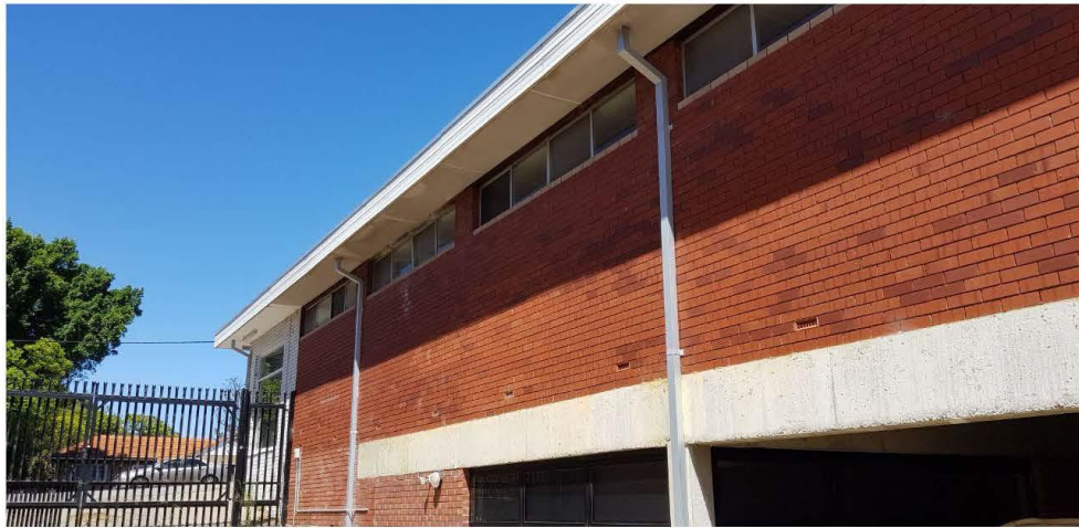
View of side of existing building
