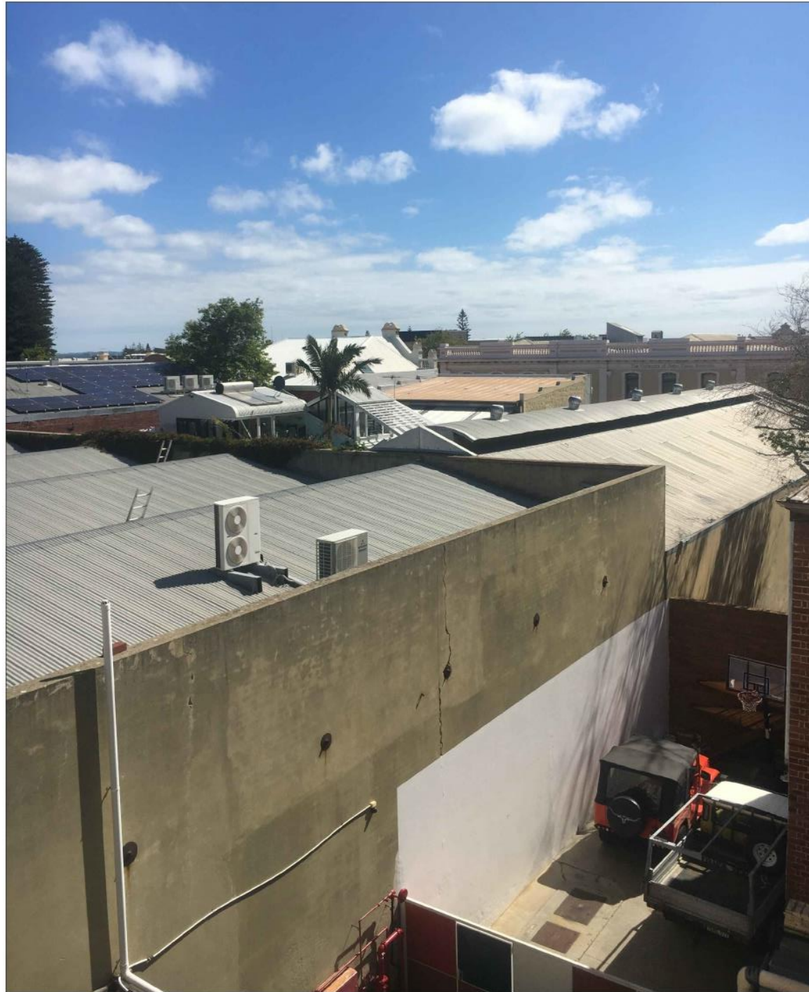
Existing view south of roof tops
