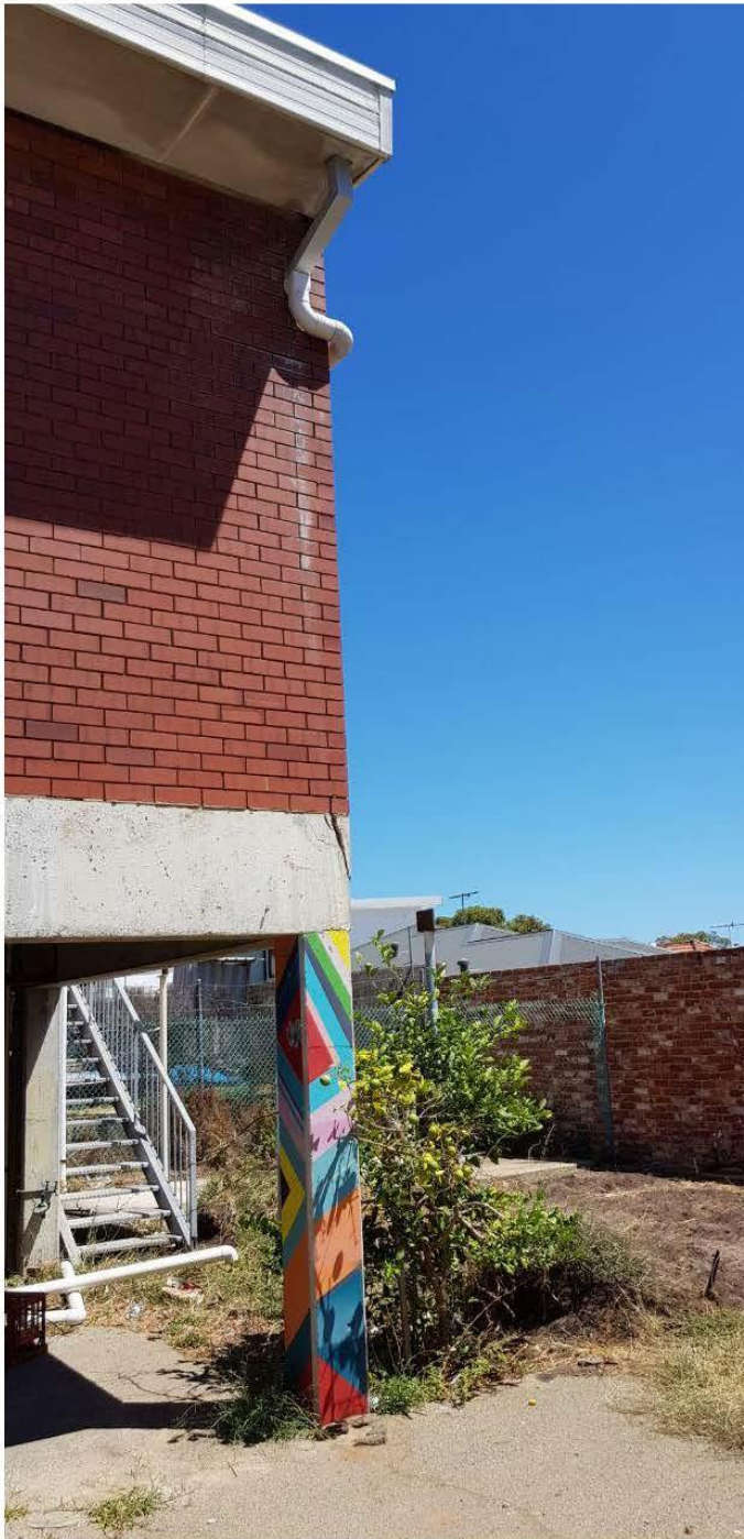
View of rear of building
