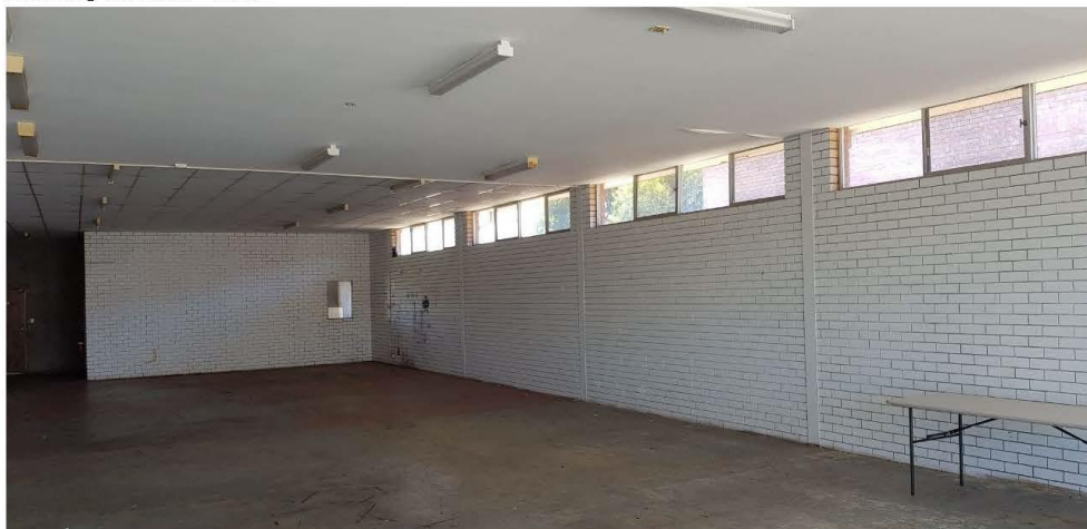
Existing internal view
