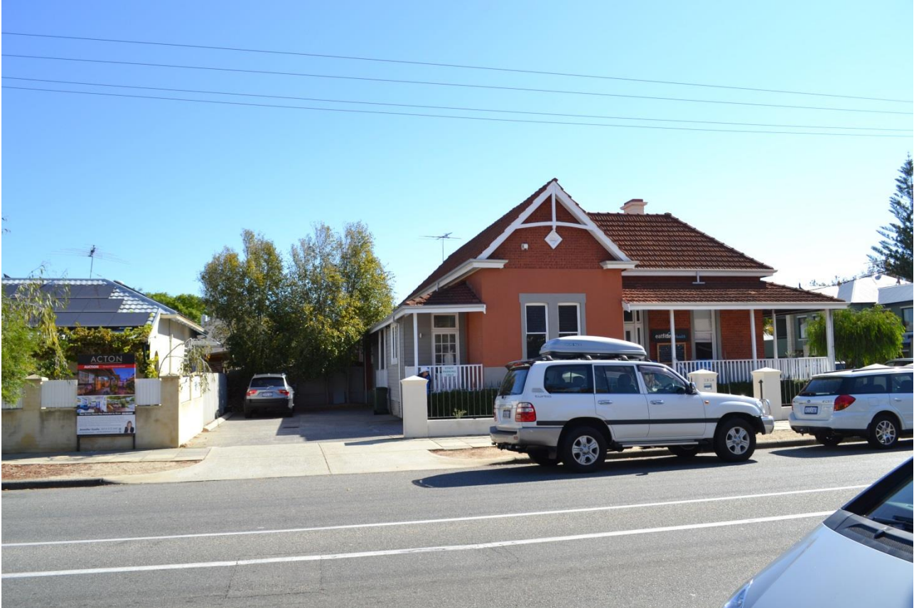
Photo 1: South Terrace streetscape of subject site and adjoining southern property.
