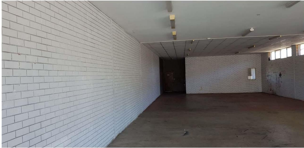
Existing internal view
