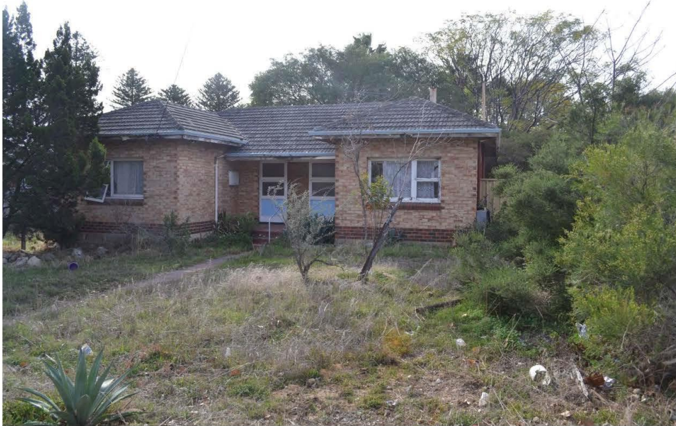
Photo 1: Existing Lefroy Road elevation
