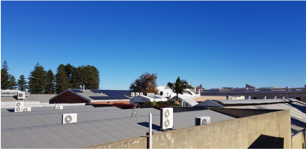
Photo 5: View over subject site facing south west
