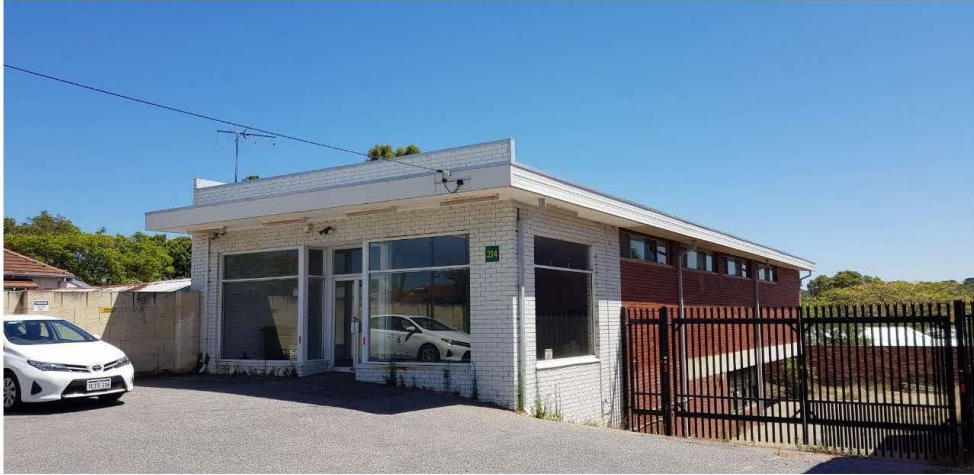
Front of existing building
