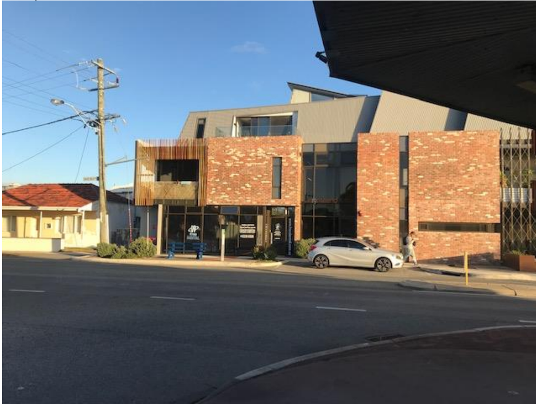
Photo 1: Northern elevation of No. 19 Douro (showing existing consulting rooms)
