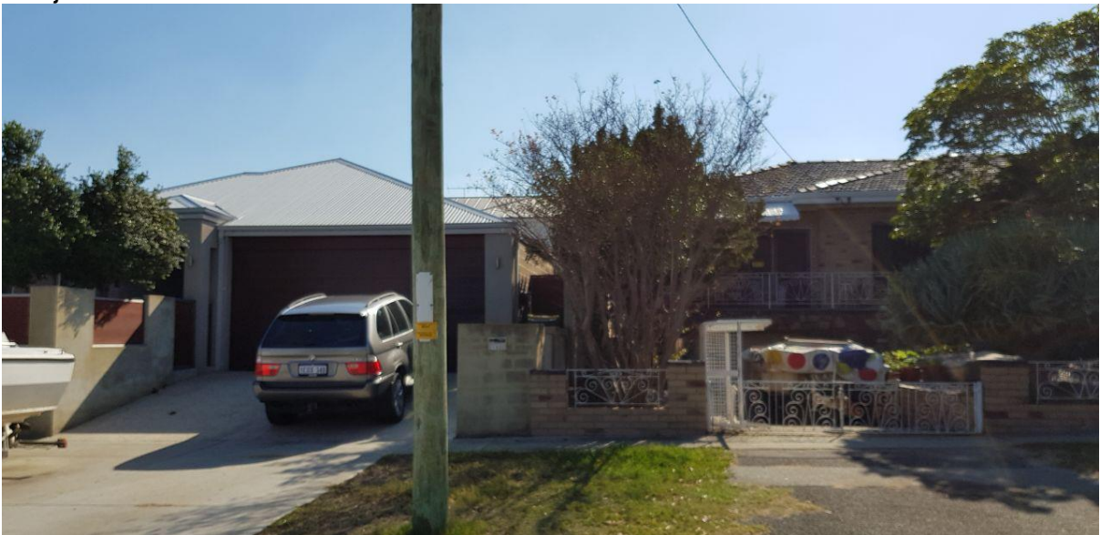
Subject site and adjoining property to west
