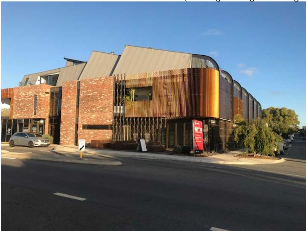
Photo 2- Intersection of Hulbert and Douro Roads (showing subject tenancy)
