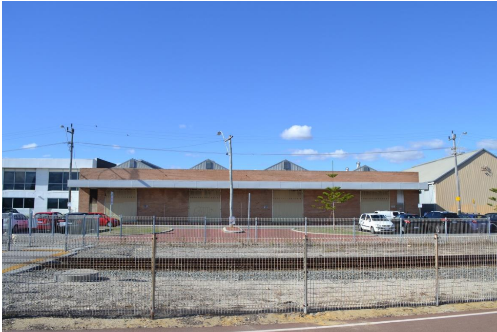
Image 5: View of Marine Terrace frontage of subject site.
