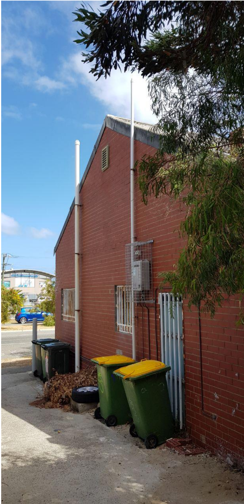
Rear of subject site
