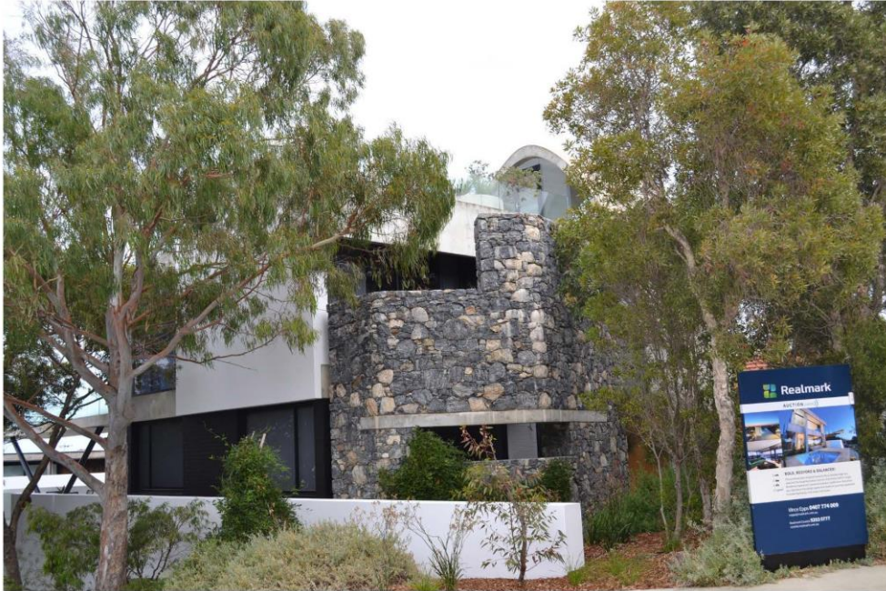
Subject site from corner Fay Street & Rule Street
