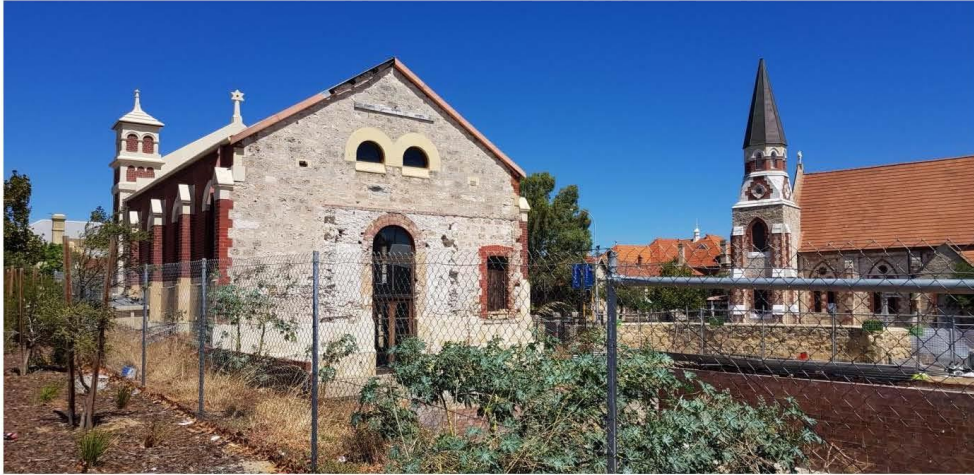
13: View of subject site from City of Fremantle car park 61 (Cappuccino Strip)
