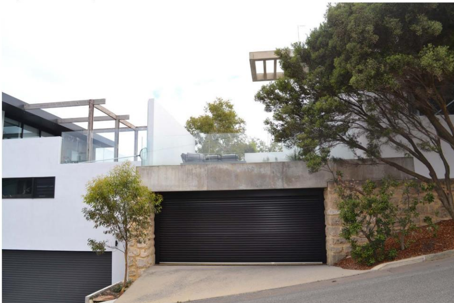
Subject site from Fay Street
