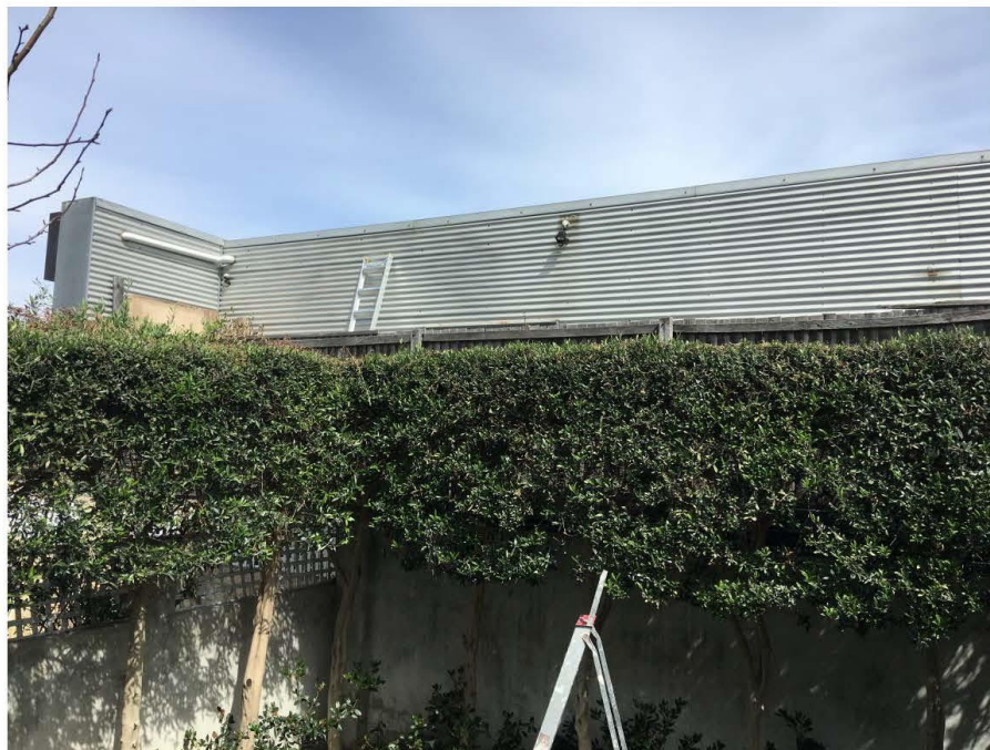
Photo 4: Northern elevation from residential lot.
