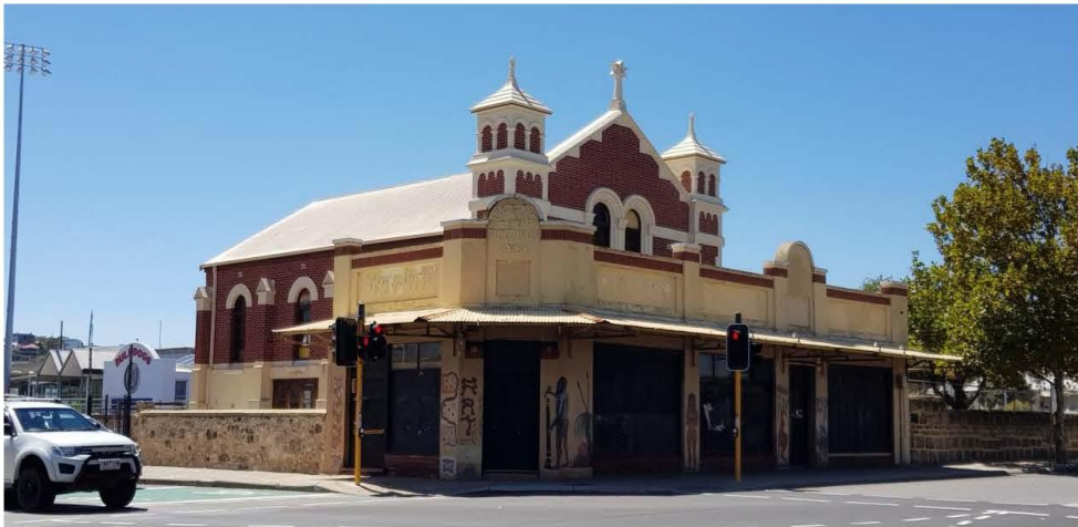
7: View of subject site from western intersection corner adjacent to Fremantle Technical College
