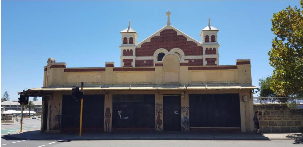
9: View of subject site from South Terrace road reserve adjacent to Norfolk Hotel
