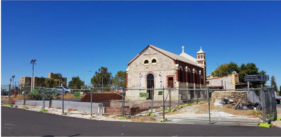
3: View of subject site from City of Fremantle Car Park 16
