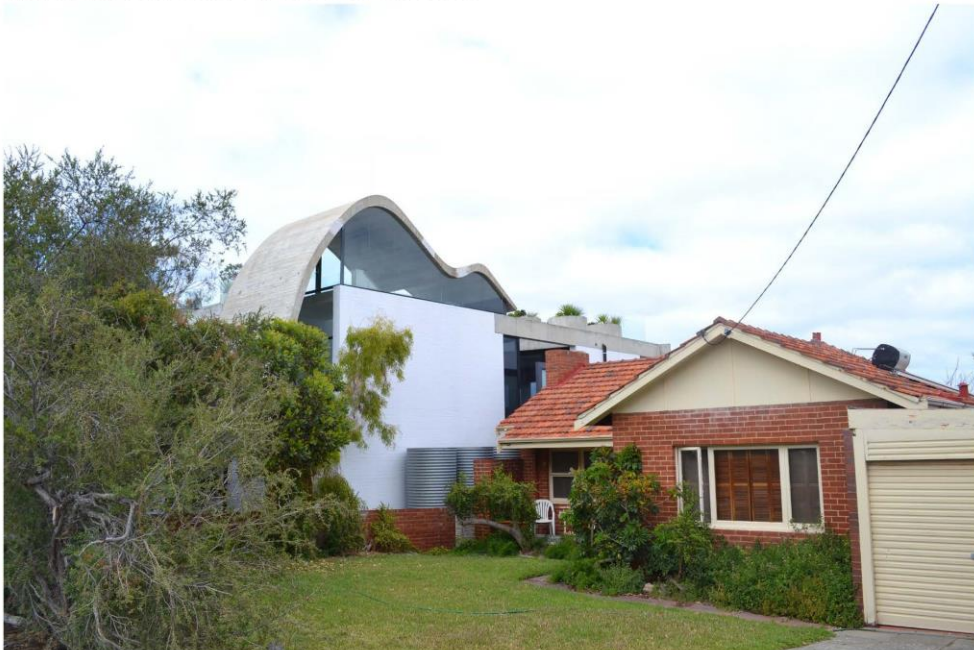
Subject site from Rule Street across the front setback of 27 Rule Street
