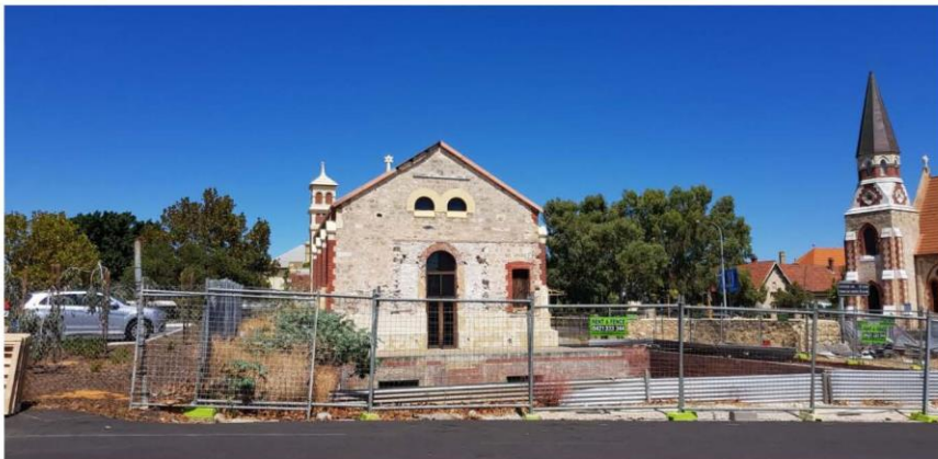
2: View of subject site from City of Fremantle Car Park 16
