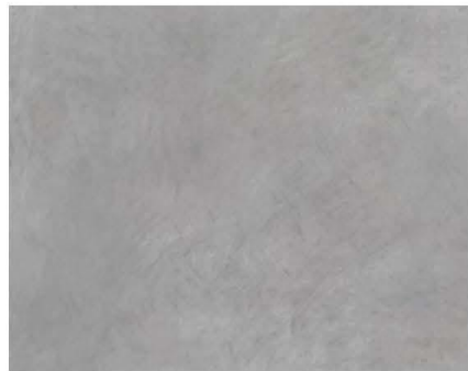
Ground level and exterior wall finish
