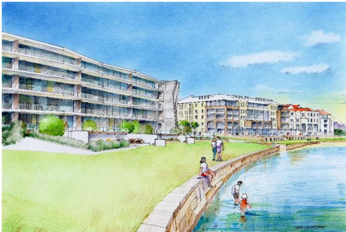
Image 1: Artist perspective of the preferred Option 1A: block wall along the riverward alignment (note: landscaping including endemic planting and paths will be developed during detailed design).
