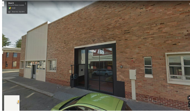
25 Mouat Street, looking south-east Source: Google Earth Streetview
