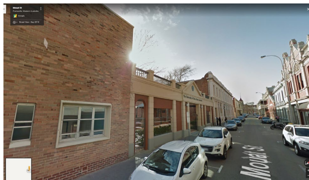
21-25 Mouat Street, looking north-west (25 to left, 23 / 21 in centre with courtyard behind)
