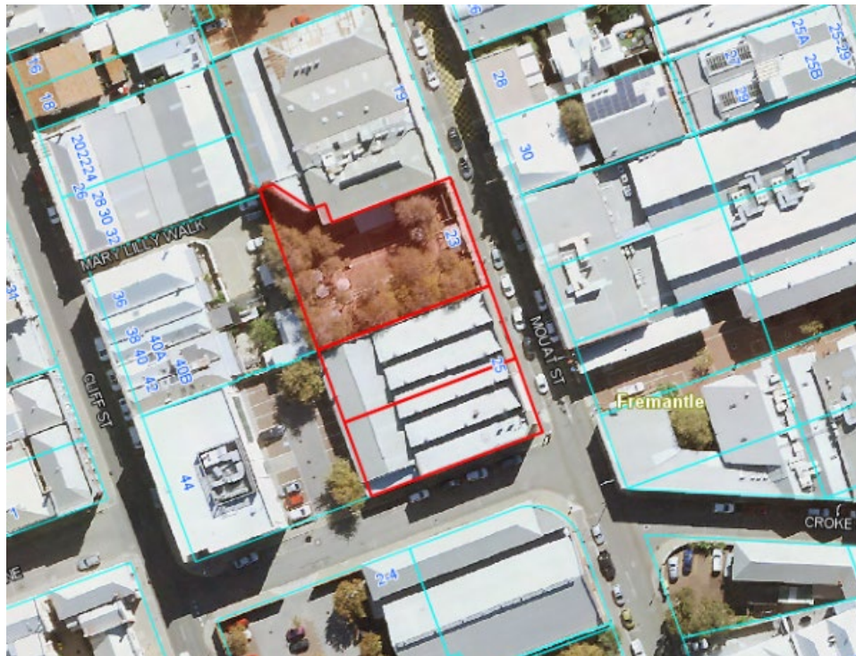
23 and 25 Mouat Street which are collectively referenced as 25 Mouat Street, Fremantle (Site of Bateman’s Warehouse) or 21-25 Mouat Street, Fremantle on the City’s heritage records
