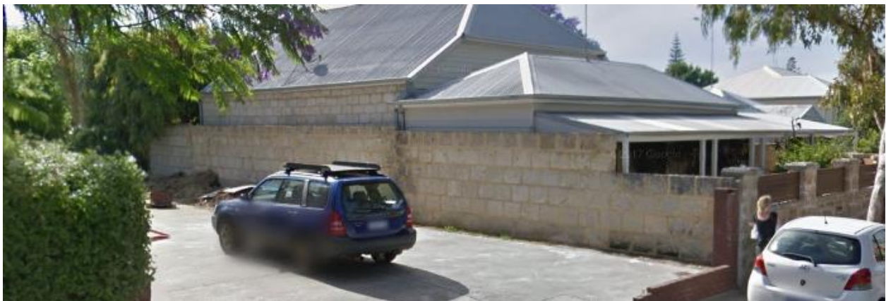
Figure 2: Adjoining boundary wall
