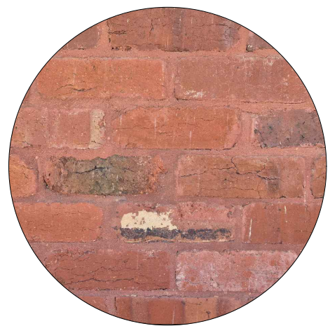
(FWK) FACE BRICKWORK NEW RECYCLED BRICKWORK TO MATCH EXISTING. GROUTING TO MATCH. WHERE POSSIBLE CLEAN & REUSE EXISTING BRICKS FROM DEMOLITION.
