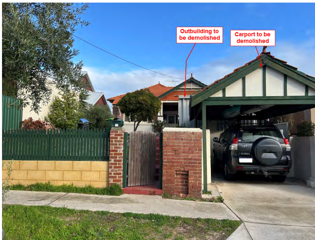
Figure 1 – Street view and structures to be demolished
