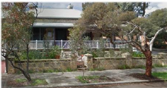
Low-scale limestone wall with piers
