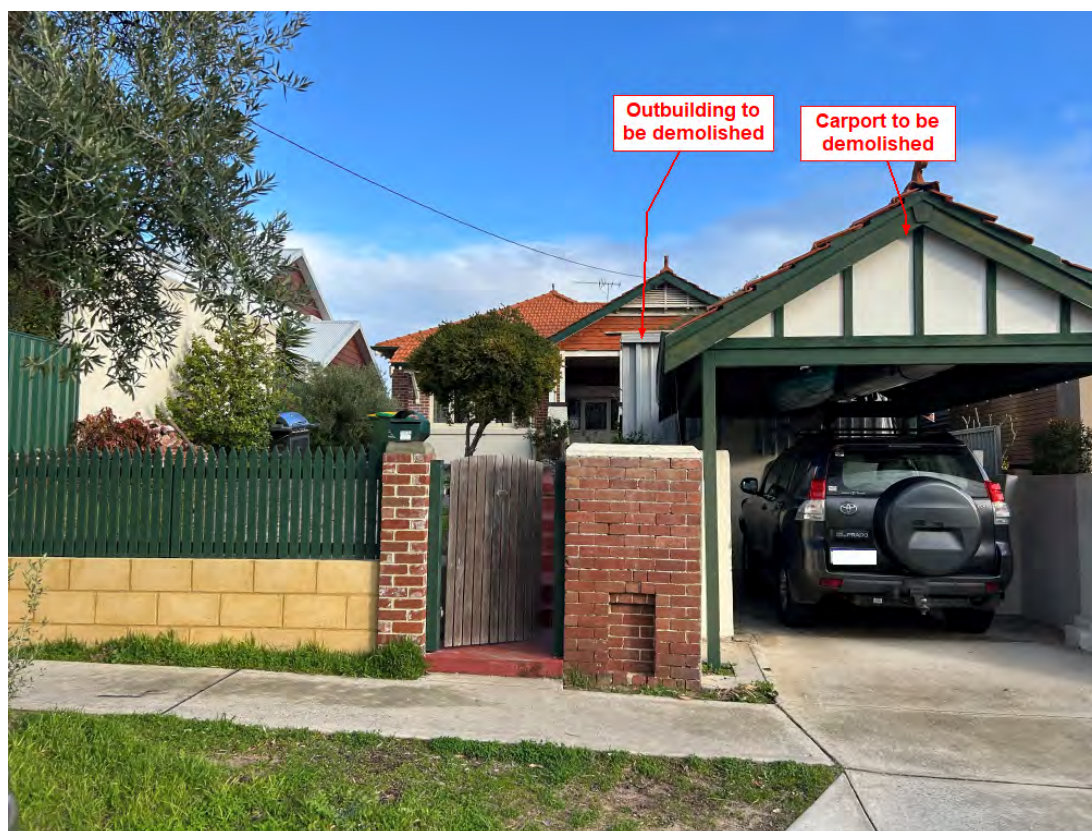
Figure 1 – Street view and structures to be demolished
