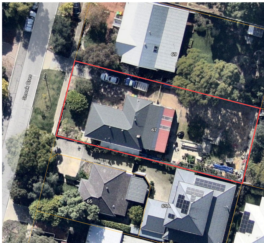
Figure 3 – Aerial image of subject site (July 2025)
