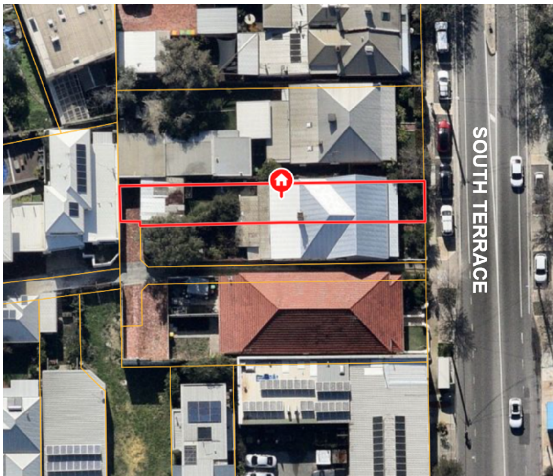
Figure 3 – Aerial image of subject site (July 2025)
