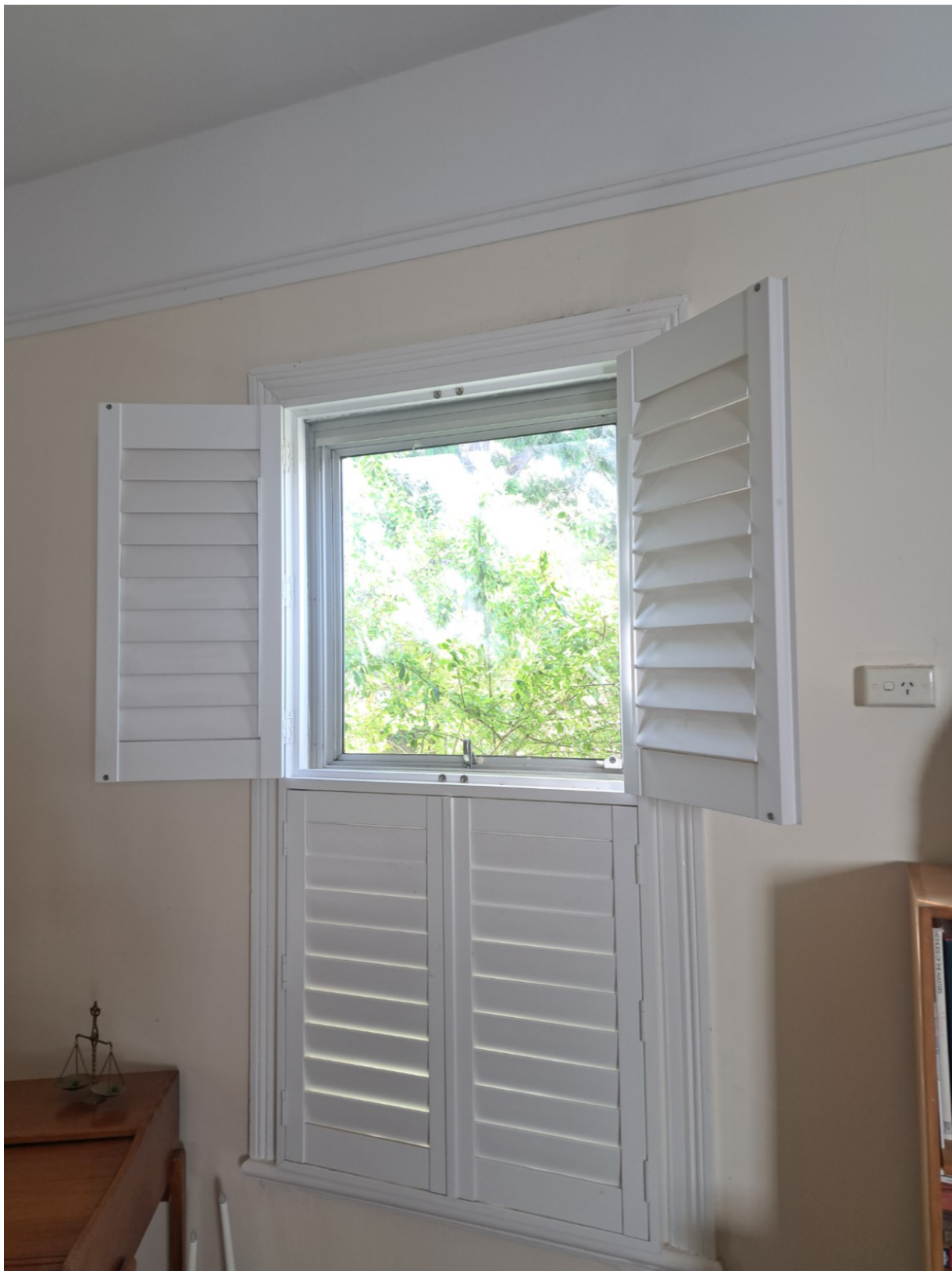
Figure 10 – impacted major opening taken from interior of impacted loungeroom of southern adjoining property with light cast at 2pm.
