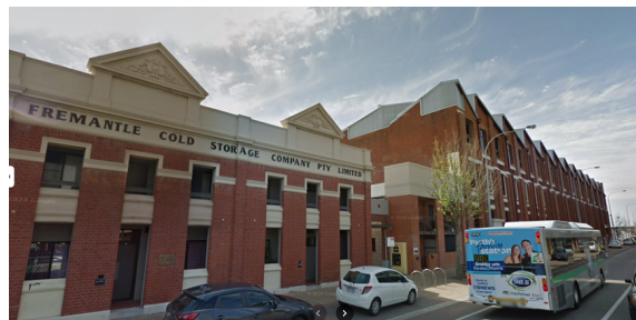
Figure 14: Area B Industrial buildings, Queen Victoria Street
