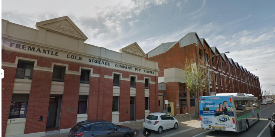
Figure 8: Area B Industrial buildings, Queen Victoria Street
