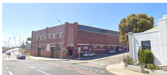
Figure 11: Area A Beach Street and James Street intersection
