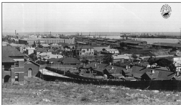
Figure 3: View of Precinct from Cantonment Hill circa 1939
