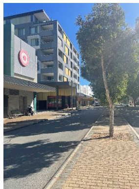
Figure 23: Contemporary streetscapes, Adelaide Street
