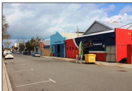
Area C Quarry Street
