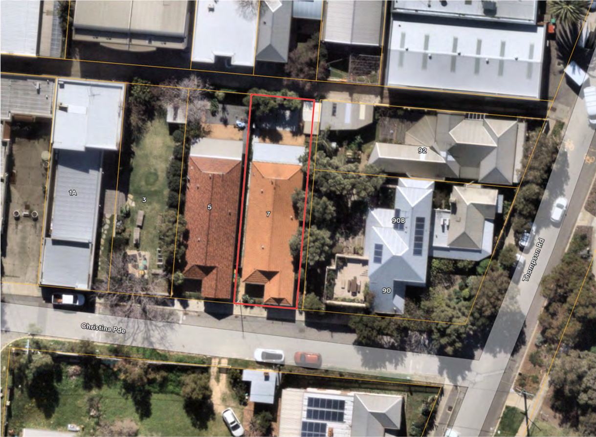
Figure 3 – Aerial image of the subject site (August 2025).
