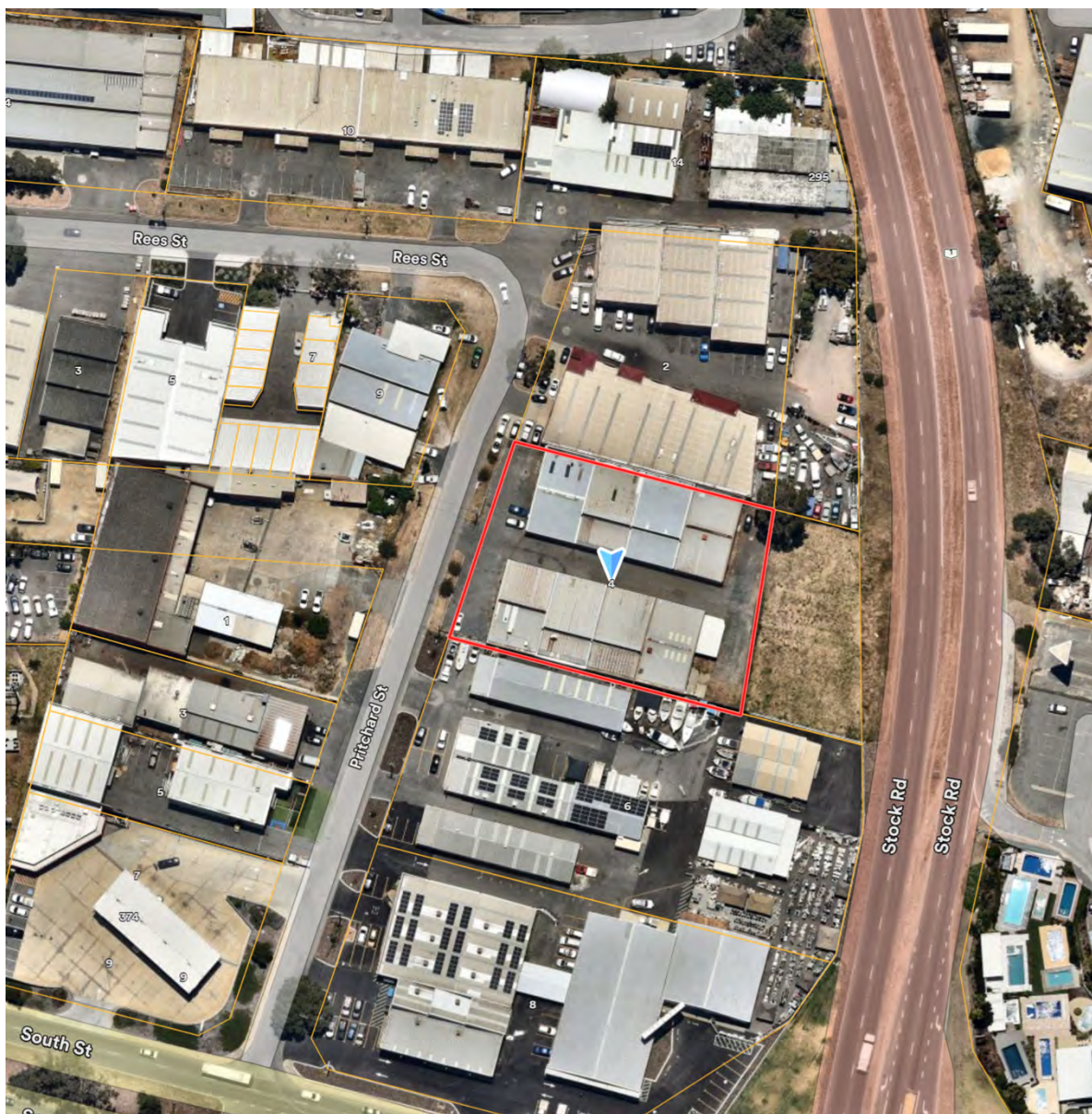
Figure 2 – Subject site aerial image (November 2025)
