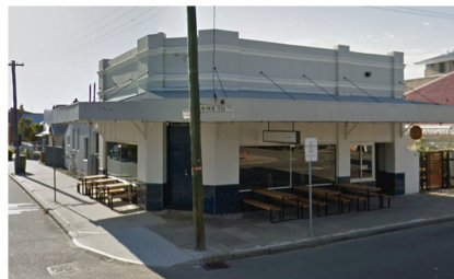
Gold-Rush era shop with Inter-War alterations to shopfronts and cantilevered awning
