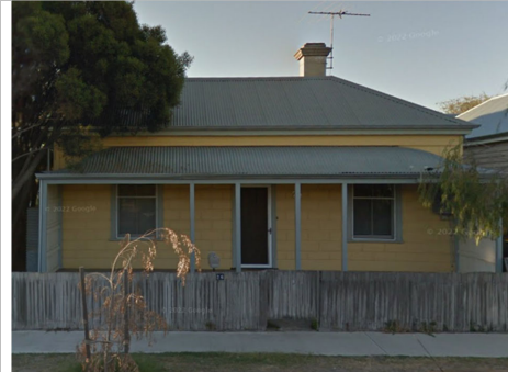
Victorian Era, typical simple four room, central corridor house
