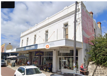
Two storey shop with residence/ storage above, North Fremantle
