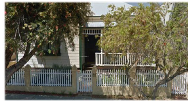
Hybrid picket and masonry front fence
