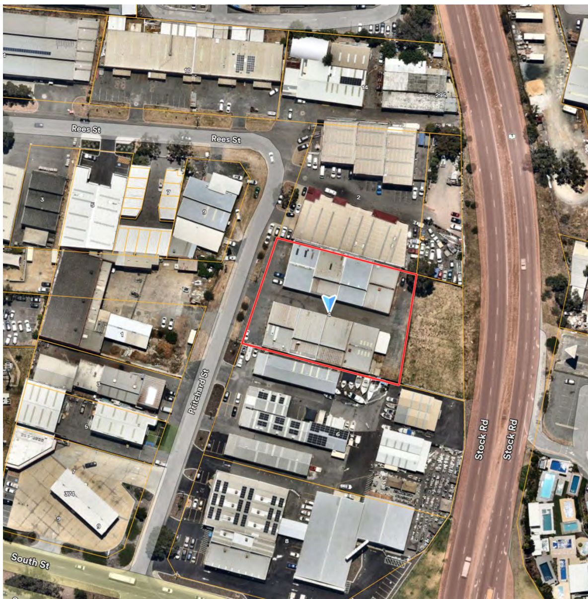
Figure 2 – Subject site aerial image (November 2025)
