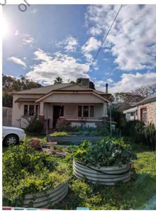
EXISTING HOUSE 56 CHESTER ST (FRONT)
