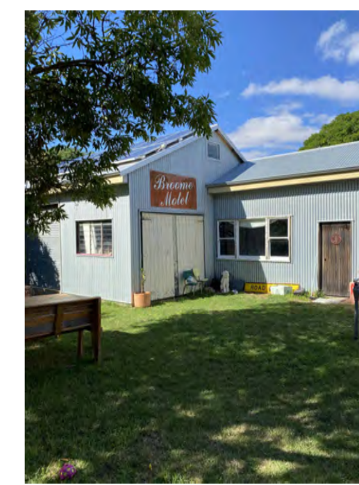
EXISTING SHED 56 CHESTER ST (FRONT)
