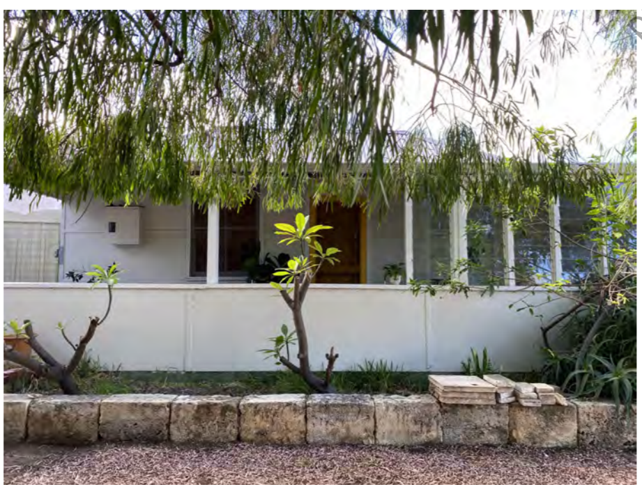
EXISTING HOUSE 54 CHESTER ST
