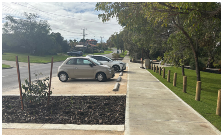
New car park and access path completed as part of the masterplan process.
