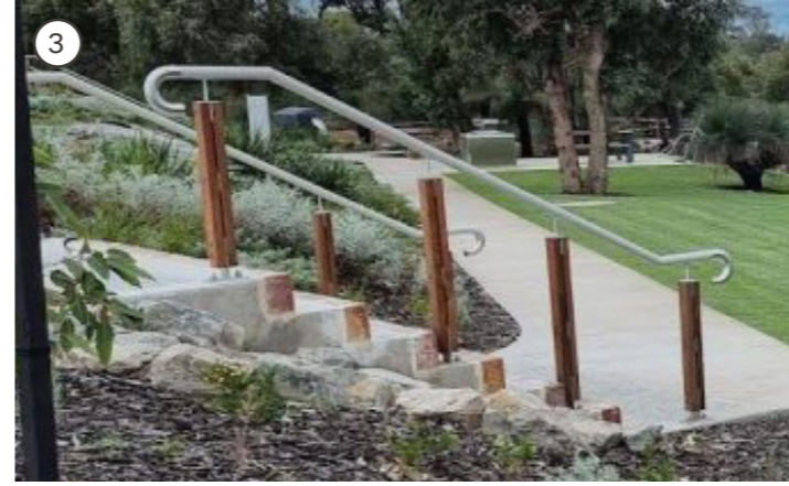
3 New landscape steps with handrails linking the carpark to an existing information hut.
