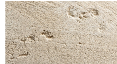
Existing limestone blocks.
